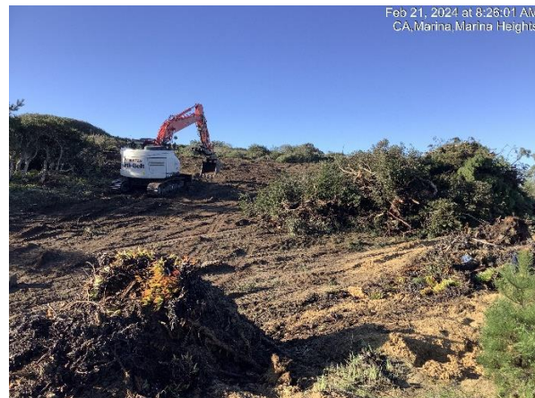
Tree & brush removal along eastbound side
