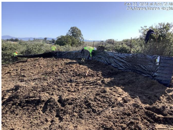
Installing perimeter silt fence
