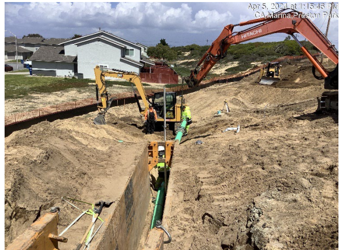
New sanitary sewer line at Preston Drive
