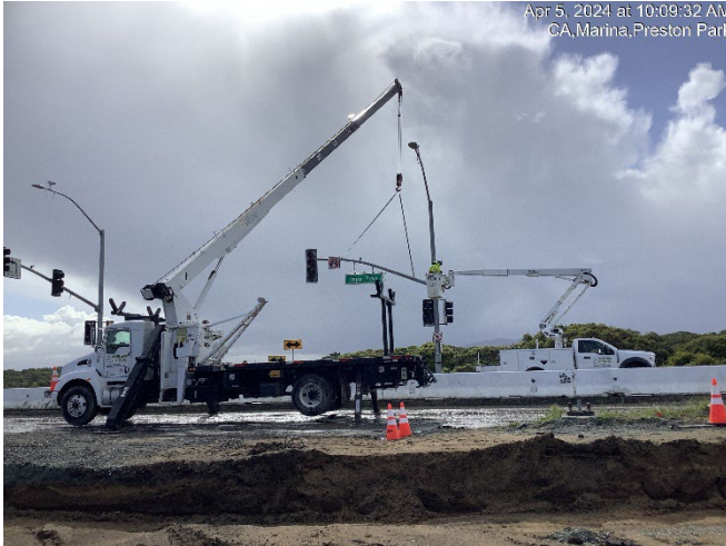
Removal of old traffic signals at Imjin Road
