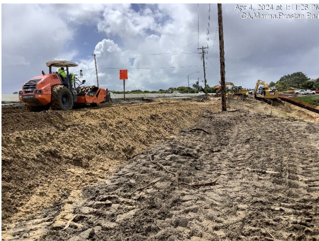
Earthwork between Reservation Road and Preston Drive
