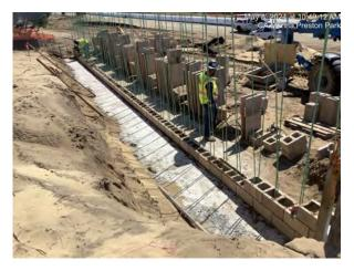
Installing concrete blocks for sound wall near Preston Park
