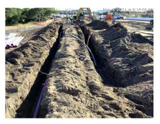
Trenching/installing irrigation service lines near Preston Park
