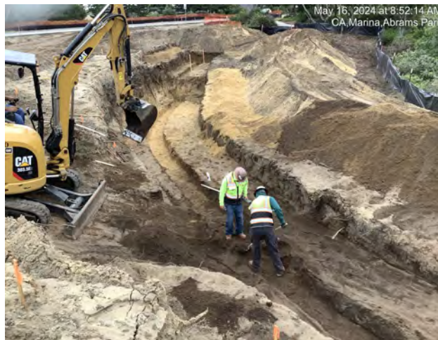
Excavation for retaining wall footing
