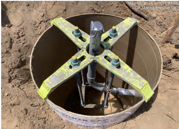
Form and bolt imbeds for street light foundation
