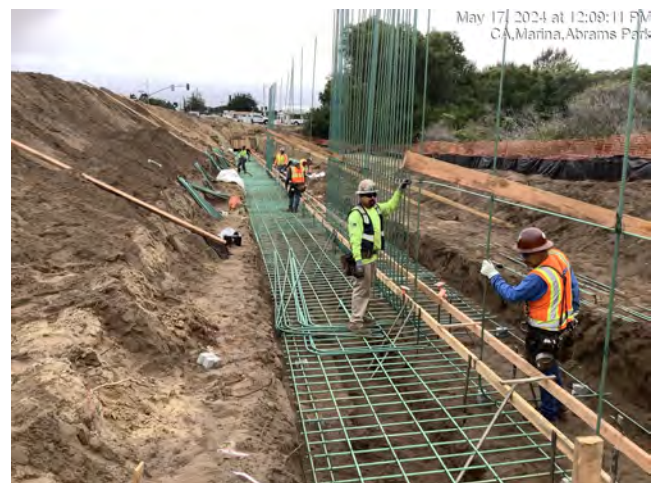
Installing bar reinforcing steel for retaining wall footing
