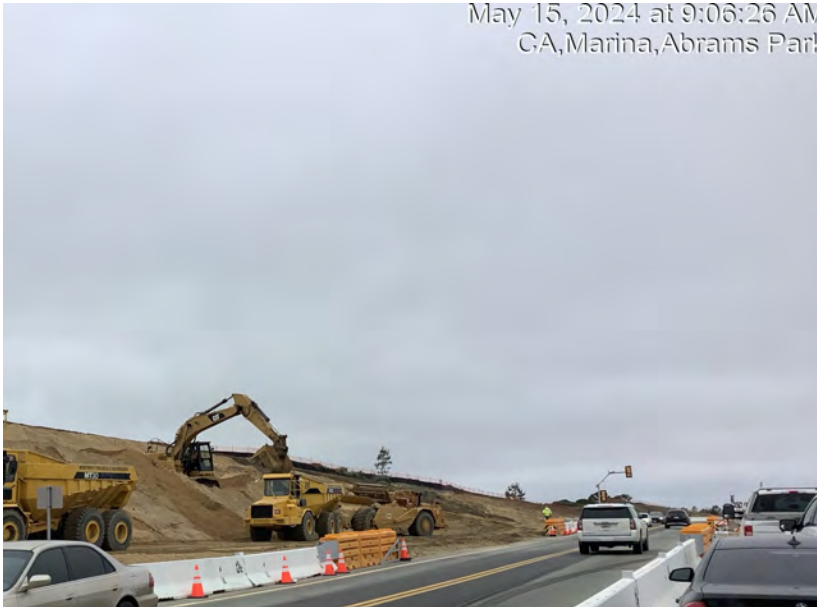
Loading trucks with dirt on south (eastbound) side to move to north (westbound) side of Imjin Parkway for use in fill operation
