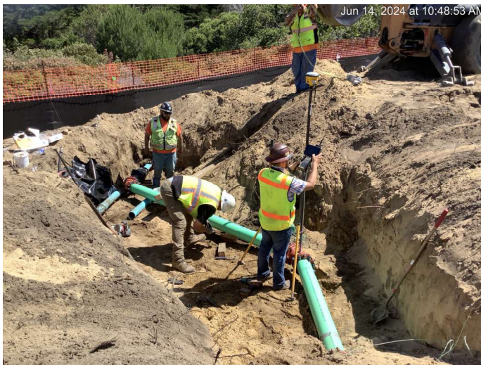
Tie-in of new 6" sewer pipe to existing line between Abrams
