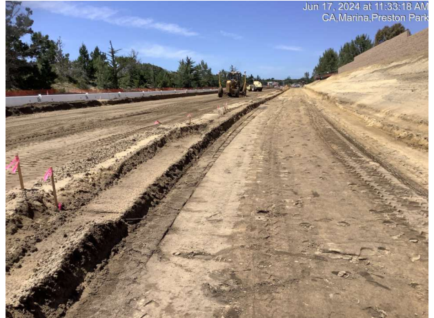
Roadway grading operations between Preston Drive and Abrams Drive
