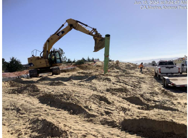
Removing abandoned sewer pipe from excavation area near Marina Heights Drive
