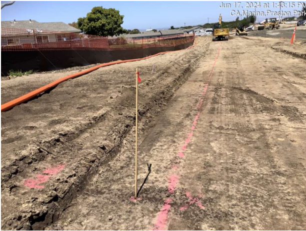
Roadway grading operations between Reservation Road and Preston Drive
