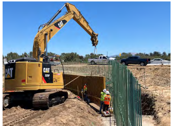
Installing form panels for the back face of retaining wall near Abrams Drive
