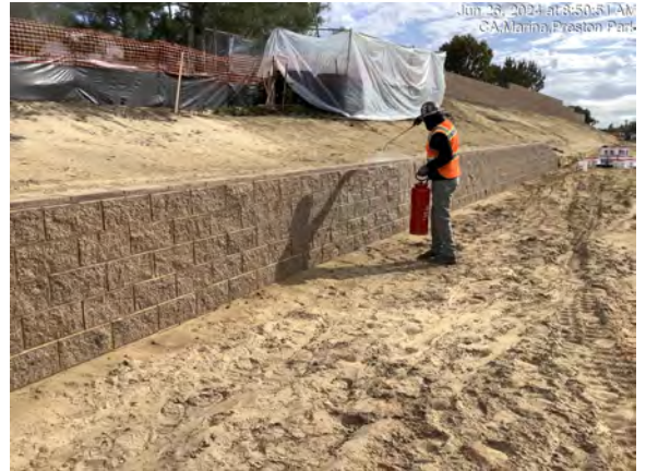
Applying anti-graffiti coating on top and face of retaining wall
