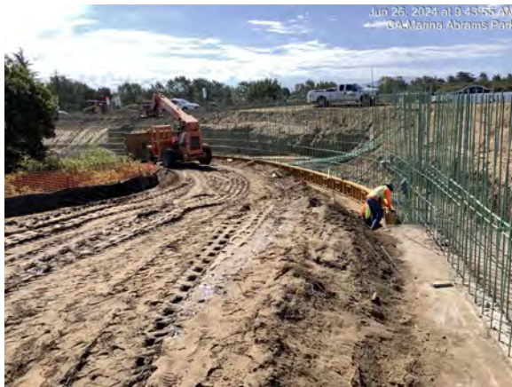
Installing form panels for the back face of retaining wall near Abrams Drive
