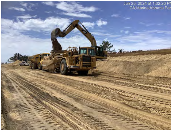
Loading material into scrapper to transport to fill slope area
