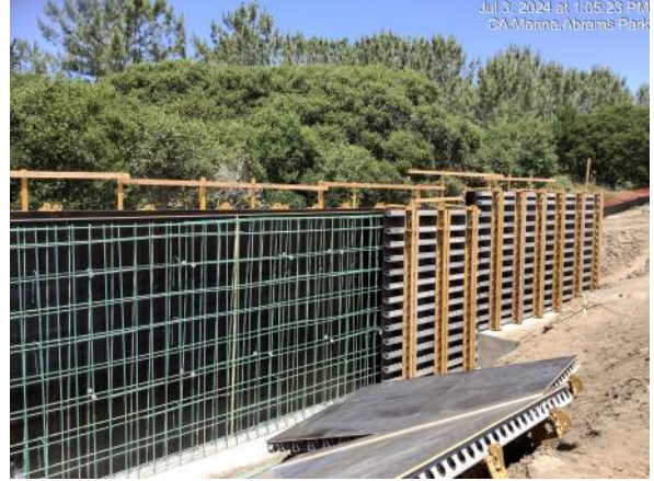
Setting forms for retaining wall near Abrams Drive
