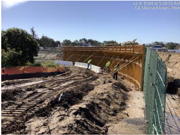
Setting forms for retaining wall near Abrams Drive
