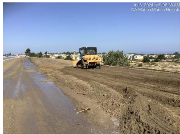
Trucks hauling dirt and equipment working spread to construct fill slope between Abrams Dr. and Preston Dr.
