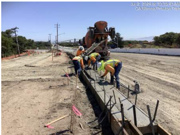
Concrete curb & gutter between Reservation Rd. & Preston Dr.
