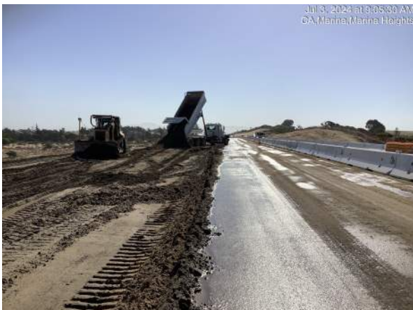
Trucks hauling dirt and equipment working spread to construct fill slope between Abrams Dr. and Preston Dr.
