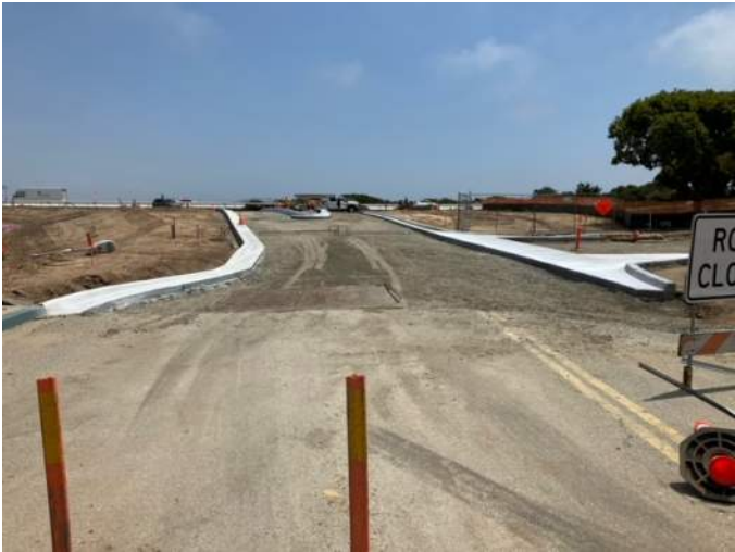
Concrete curb & gutter on new Preston Drive
