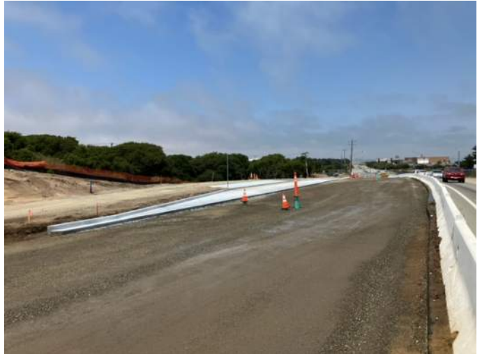
Concrete curb & gutter and bus pad on new Imjin Parkway
