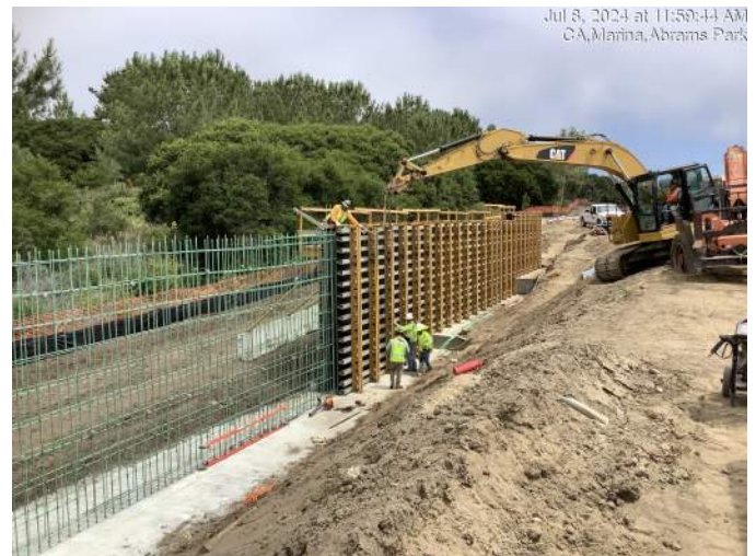
Assembling formwork for retaining wall near Abrams Drive
