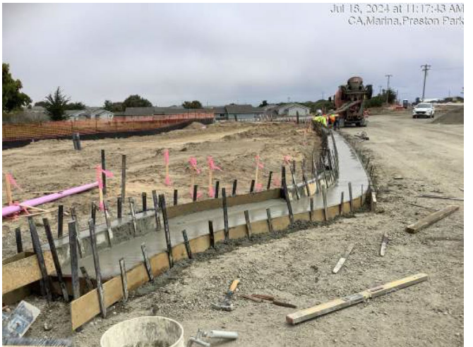
Concrete work for curb and gutter along Imjin Parkway west of Preston Drive
