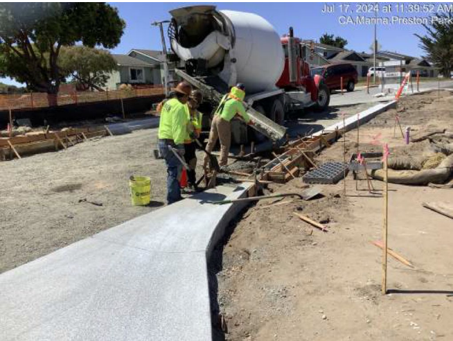
Concrete work for curb and gutter along Imjin Parkway west of Preston Drive
