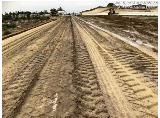
Importing fill material and grading to construct fill slopes between Abrams Drive and Marina Heights Drive
