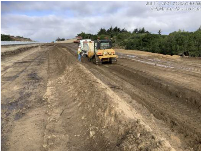
Importing fill material and grading to construct fill slopes between Abrams Drive and Marina Heights Drive
