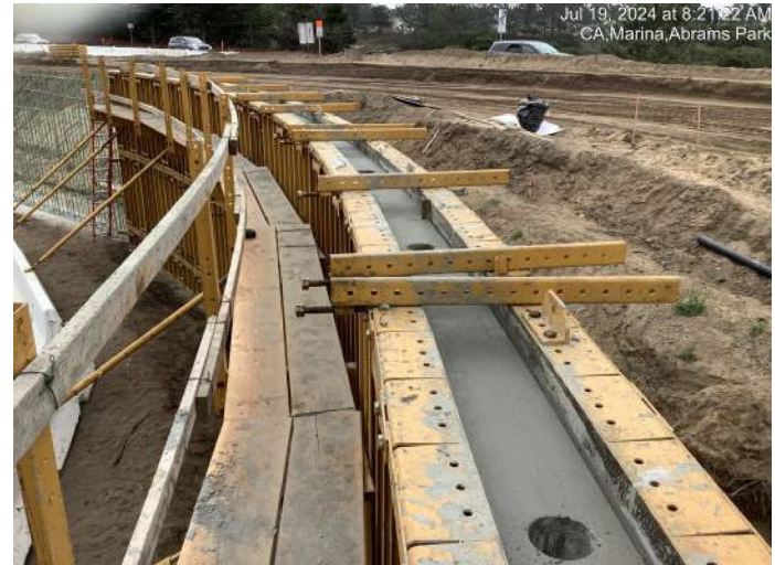
Top of retaining wall with post hole pockets for future railing
