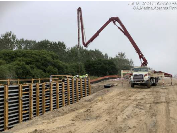
Pumping concrete into retaining wall forms (near Abrams Dr.)
