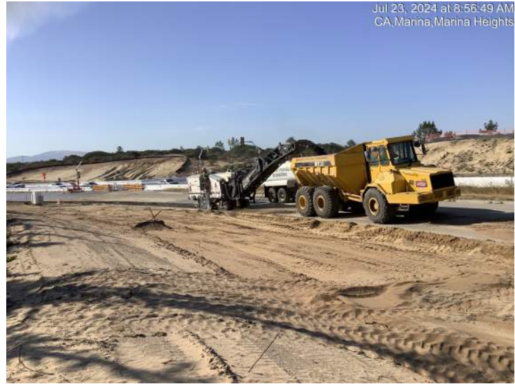
Pavement grinding operation west of Marina Heights Drive
