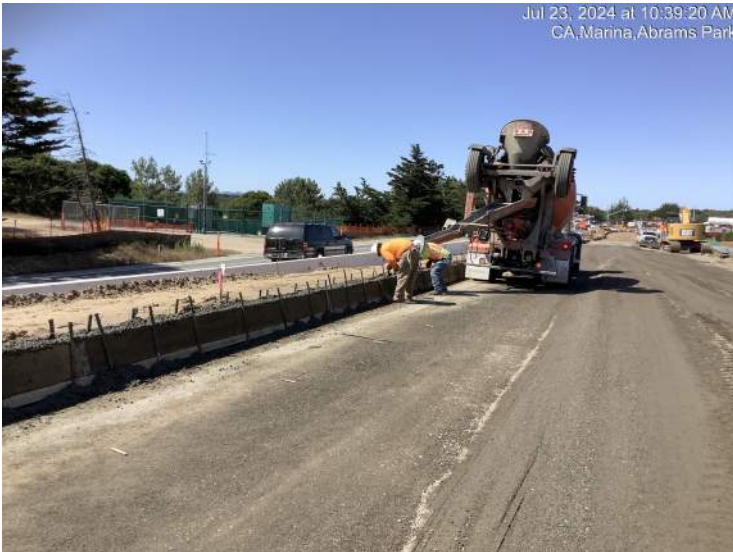
Concrete being placed for median curbs along Imjin Parkway
