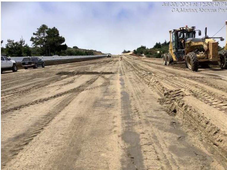
Grading for bike path adjacent to roadway section
