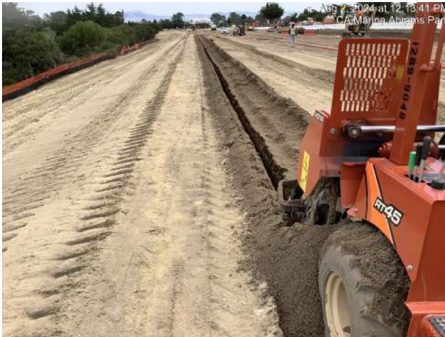
Trenching and installing fiber optic cable west of Abrams Drive
