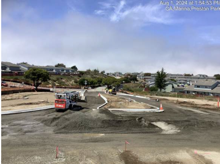
Installing base material for roadway section on Preston Drive
