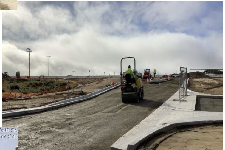
Compacting base material for roadway section on Preston Drive
