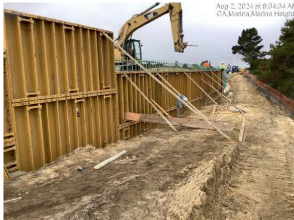
Installing forms for back of retaining wall near Marina Heights Drive
