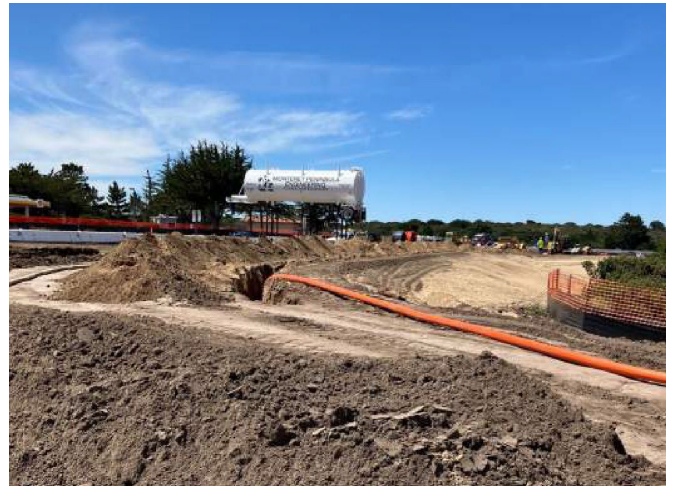
Trenching and installing fiber optic cable west of Abrams Drive
