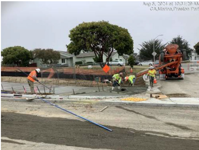
Forming and concrete finishing for new sidewalks on Preston Drive
