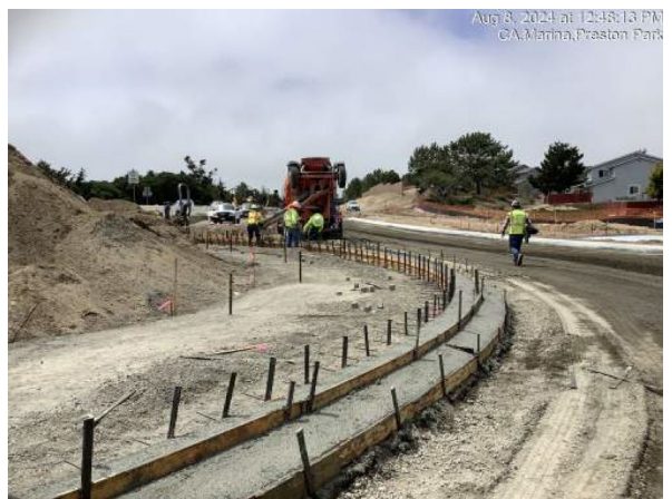
Forming and concrete finishing for new sidewalks on Preston Drive
