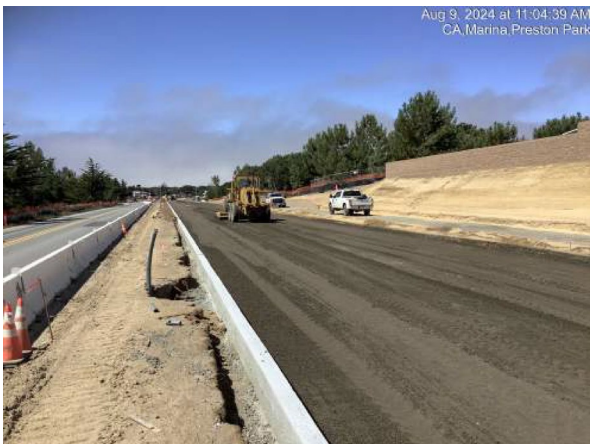
Fine grading operations for roadway section in preparation for paving from Reservation Road to the west of Preston Drive
