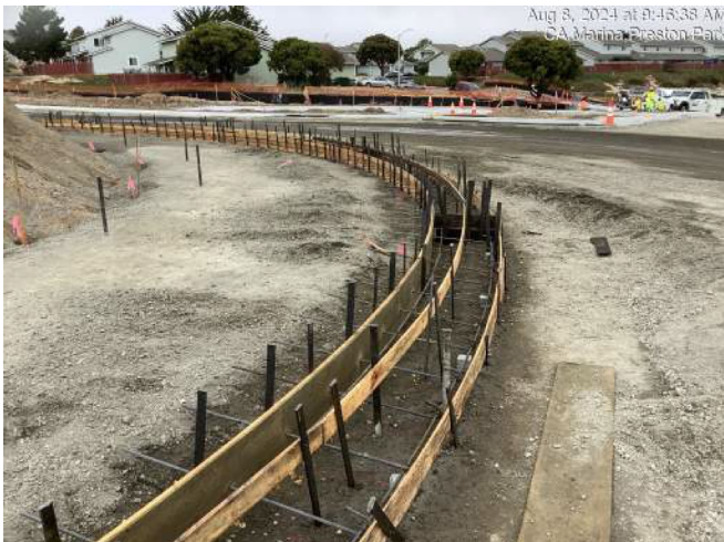
Forming and concrete finishing for mountable truck curb @ Preston Drive roundabout
