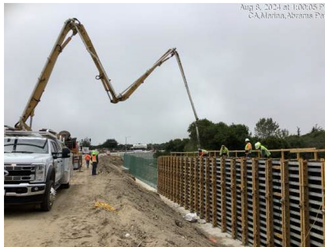
Concrete pump delivering concrete for retaining wall near Preston Drive
