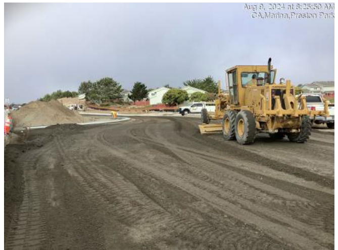
Fine grading operations for roadway section in preparation for paving from Reservation Road to the west of Preston Drive
