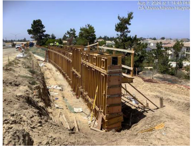
Setting forms for concrete retaining wall sections near Marina Heights Drive
