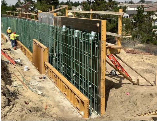
Setting forms for concrete retaining wall sections near Marina Heights Drive
