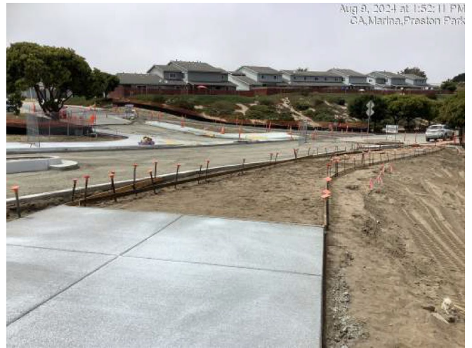
Forming and concrete finishing for new sidewalks on Preston Drive
