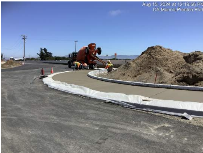
Concrete for truck apron at roundabout for Preston Drive
