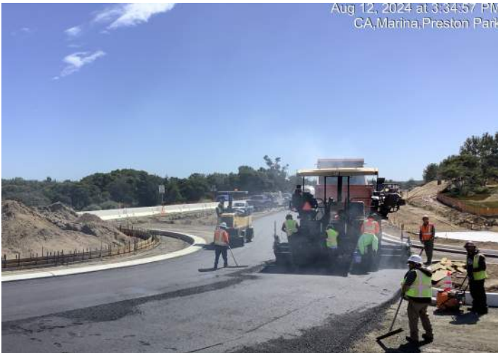
Paving operation at top of Preston Drive
