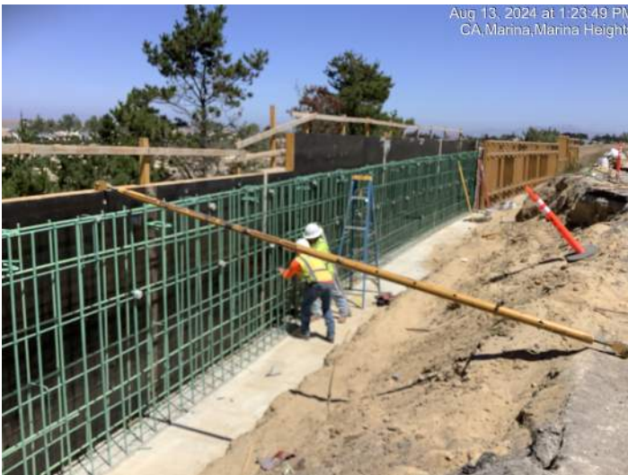
Striping and resetting retaining wall forms near Marina Heights Drive
