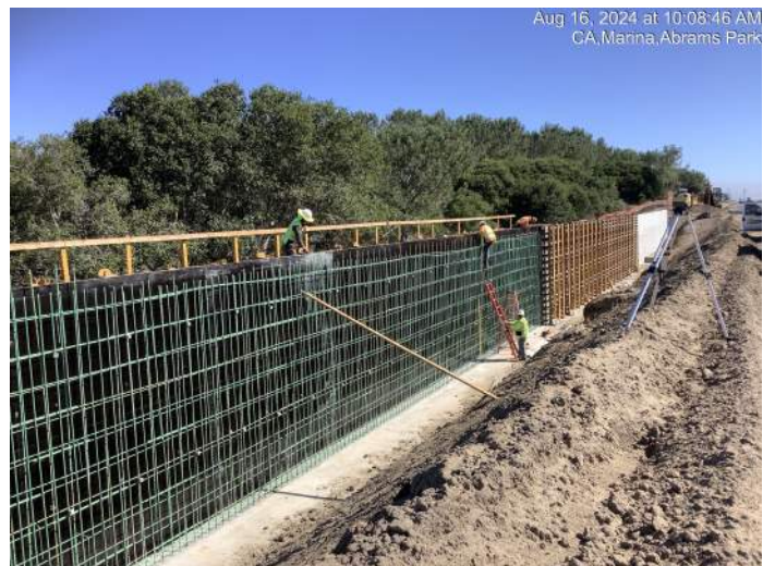
Striping and resetting retaining wall forms near Abrams Drive
