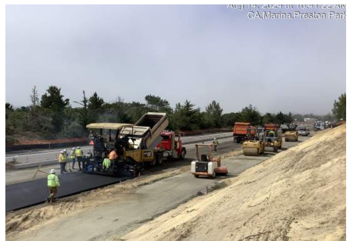
Paving operation west of Preston Drive
