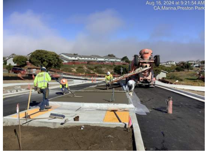
Median concrete placement along Preston Drive
