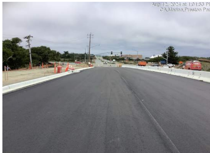
First layer of asphalt pavement between Preston Drive and Reservation Road
