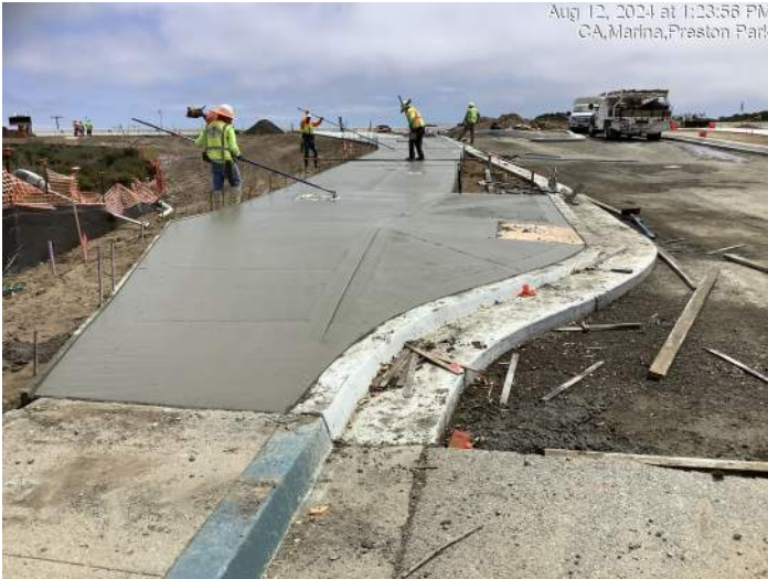
Sidewalk and ramp concrete along Preston Drive
