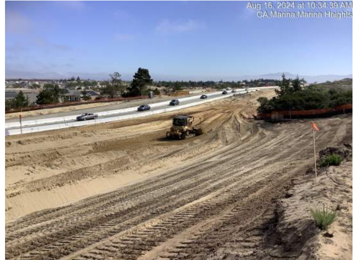
Earthwork continues near Marian Heights Drive
