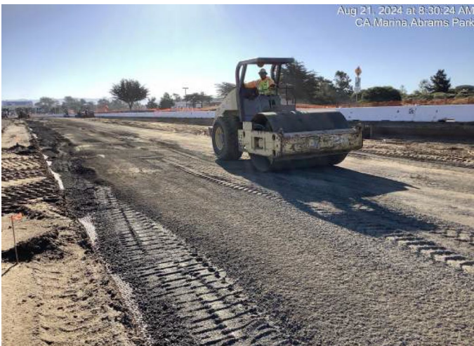
The roadway design includes the use of "geo-grid" which adds strength and stability to the material beneath the asphalt surface
