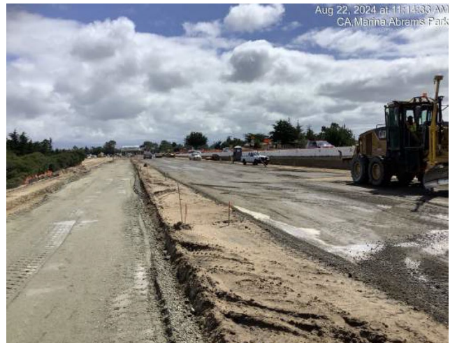
"Base rock" is installed on top of the geo-grid and is graded, then compacted. Asphalt will be the final layer on top of the base rock section.
