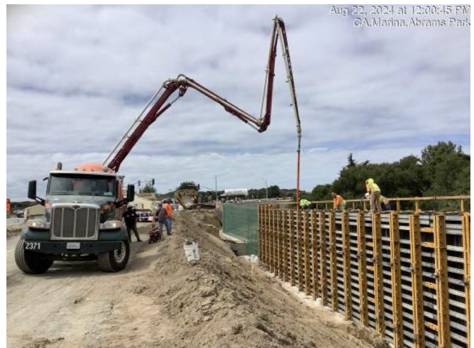
Concrete pump delivering concrete for the retaining wall near Abrams Drive.
