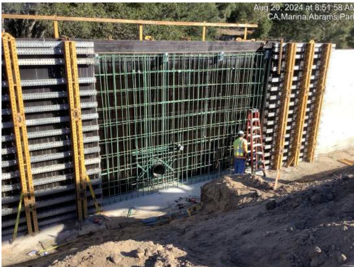
Resetting forms for the concrete retaining wall near Abrams Drive.
