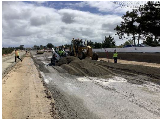
"Base rock" is installed on top of the geo-grid and is graded, then compacted. Asphalt will be the final layer on top of the base rock section.
