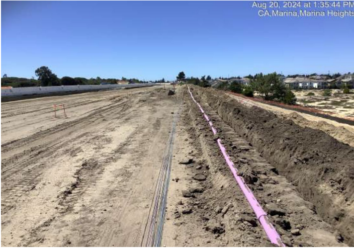
Trenching for irrigation service lines. Purple pipe is for recycled water use.
