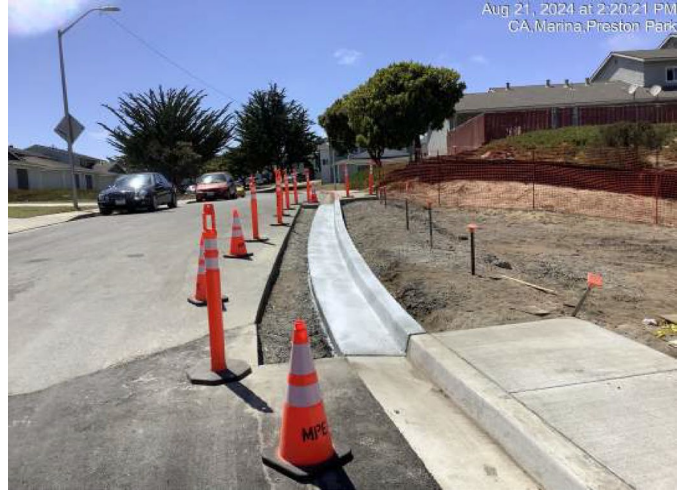
Curb and gutter work at Ready Court
