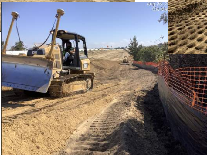
Earthwork operations for fill slopes between Abrams Drive and Imjin Road
