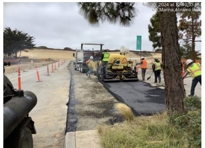
Median removal and temporary paving at the top of Marina Heights Drive
