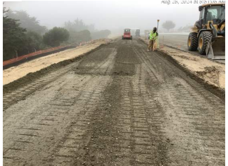
Installation of base materials for the bike path adjacent to new Imjin Parkway roadway
