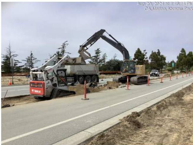
Median removal and temporary paving at the top of Marina Heights Drive
