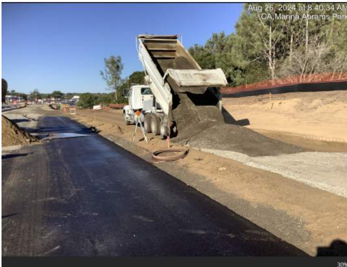
Installation of base materials for the bike path adjacent to new Imjin Parkway roadway
