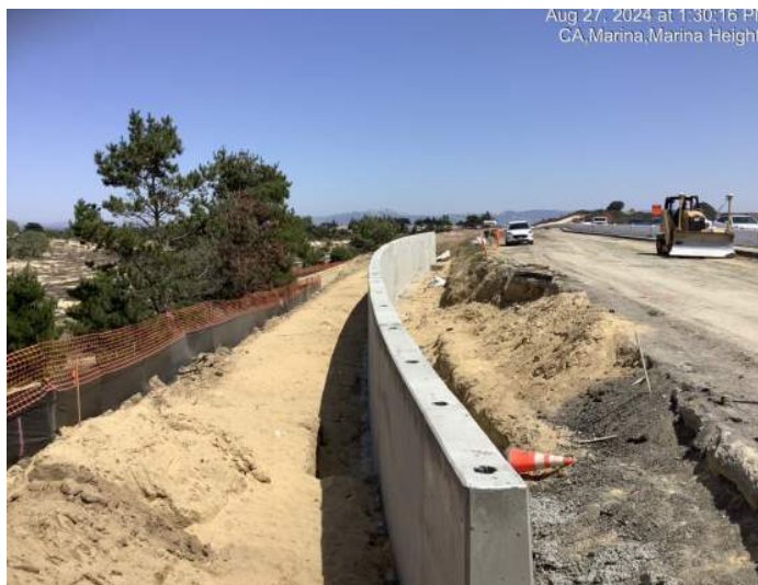
Concrete retaining wall near Marina Heights Drive completed
