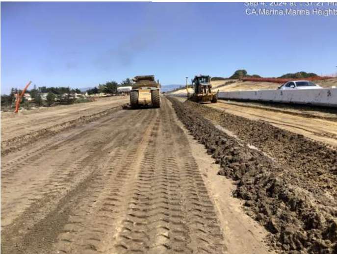
Earthwork/grading between Abrams Drive & Marina Heights Drive
