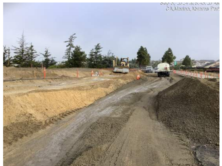
Earthwork/grading operations on Marina Heights Drive
