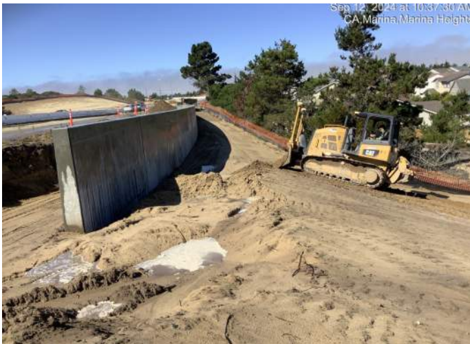
Backfilling operations at concrete retaining wall near Marina Heights Drive
