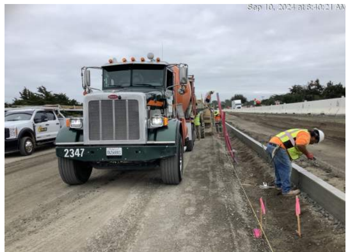
Finishing touches on the extruded concrete curb
