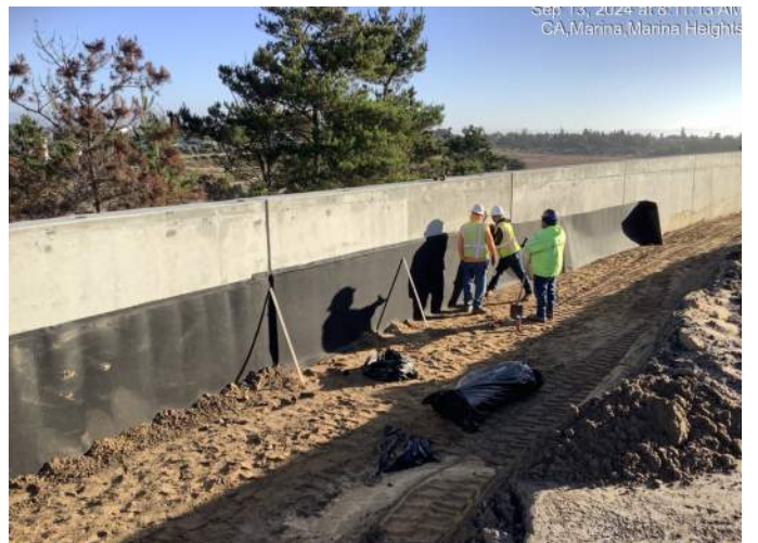
Installing geotextile material on roadway side of concrete retaining wall near Marina Heights Drive.
