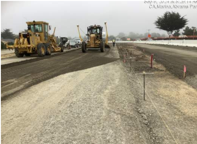
Grading and compaction activities on roadway section between Abrams Drive and Marina Heights Drive
