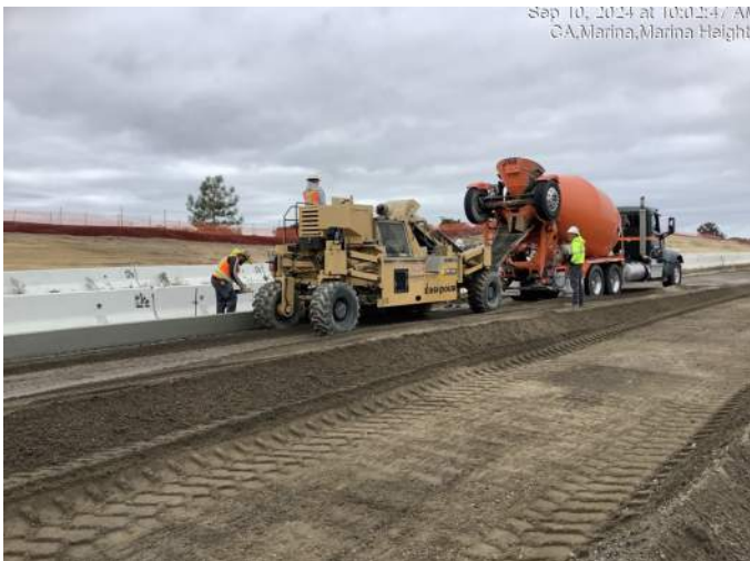
Concrete extrusion machine receives concrete in the front and molds/places concrete for median curb
