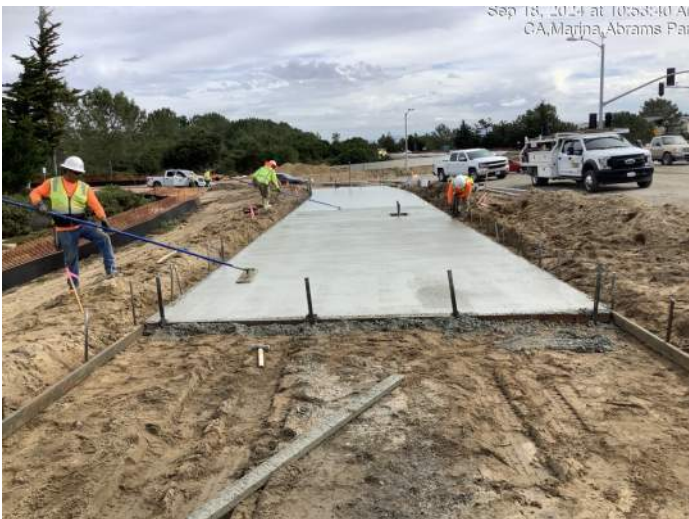
Finishers working on sidewalk/path concrete near Abrams Drive
