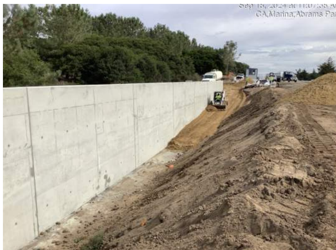
Backfilling concrete retaining wall near Abrams Drive
