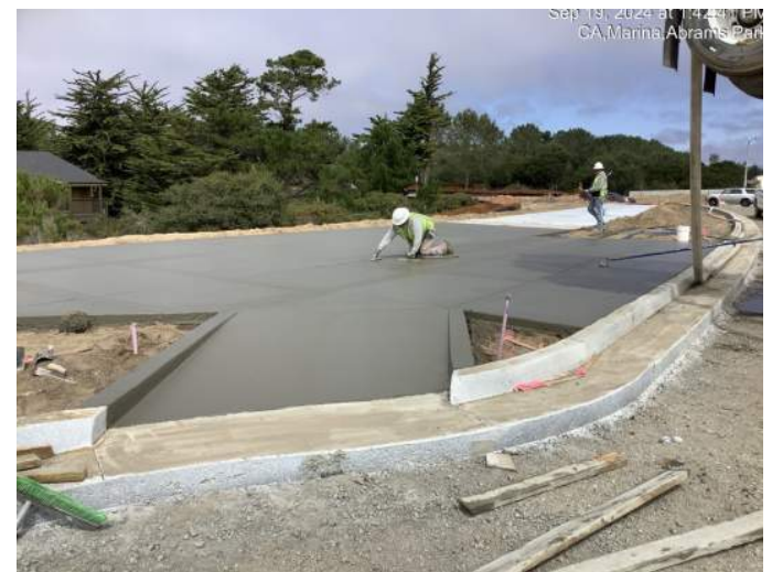
Finishers working on sidewalk/path concrete near Abrams Drive
