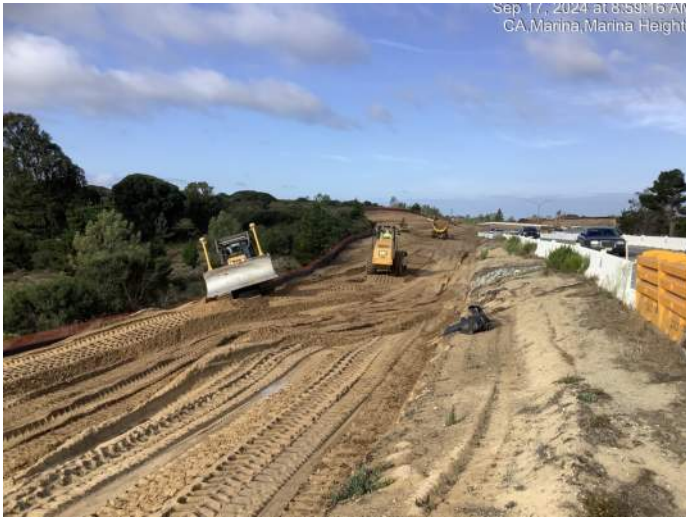
Earthwork to construct fill slope on south side of Imjin Parkway
