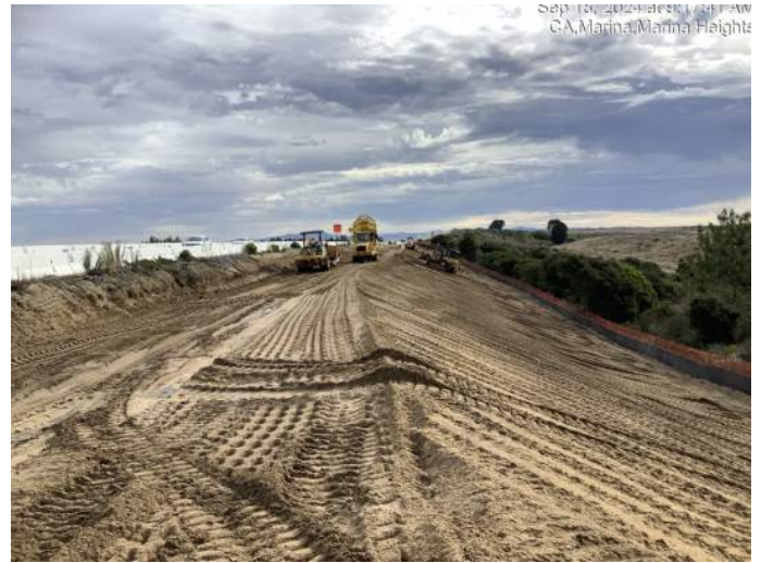
Earthwork to construct fill slope on south side of Imjin Parkway
