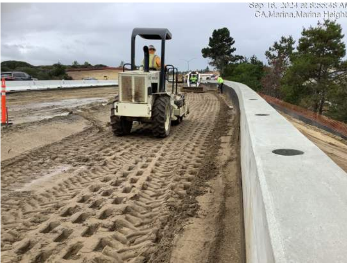
Backfilling nearly complete at retaining wall near Marina Heights Drive
