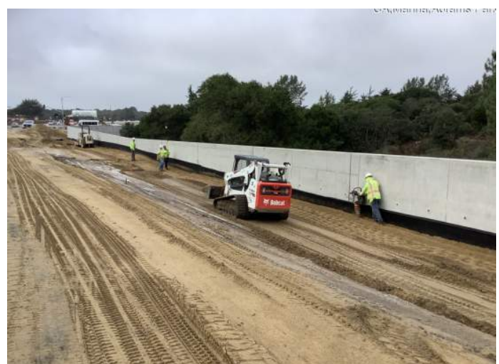
Backfilling concrete retaining wall near Abrams Drive
