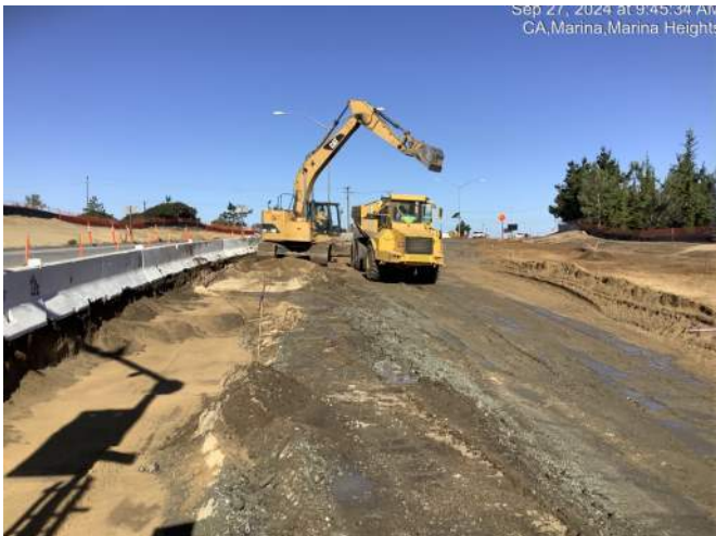
Earthwork along Imjin Parkway west of Imjin Road
