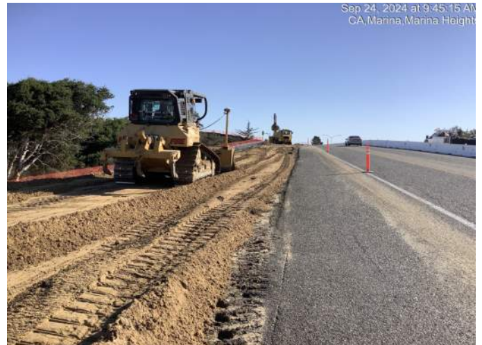
Grading along west side of Imjin Road
