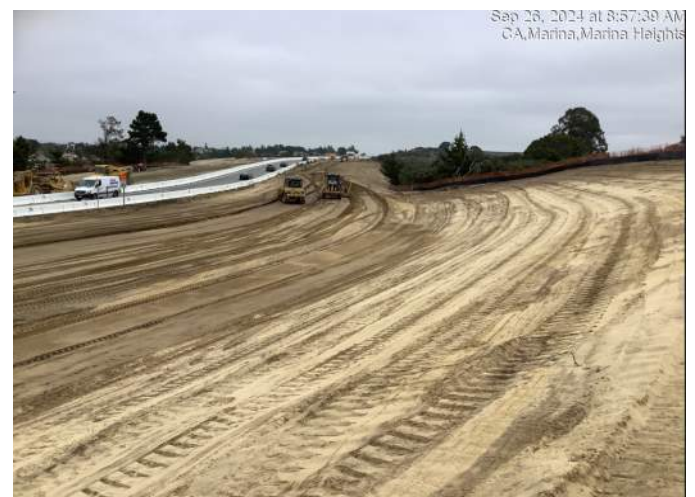
Embankment grading along Imjin Parkway east of Imjin Road
