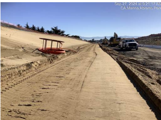
Grading for bike path between Abrams Drive & Marina Heights Drive
