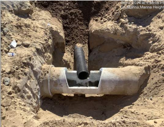
Installing new storm drain into existing drainage system.
