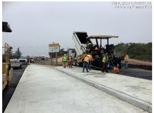
Paving bike path between Reservation Rd and Preston Dr
