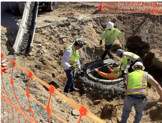
Placing a concrete manhole base for storm drain at Imjin Road
