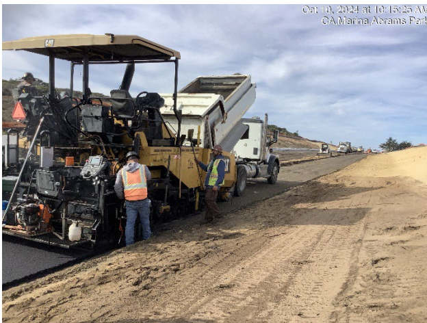
Paving first lift of roadway between Abrams and Marina Heights
