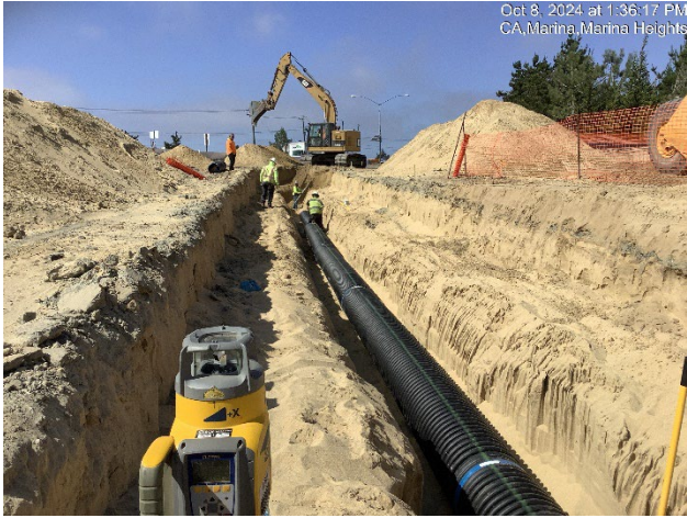
Placing storm drain pipe at Imjin Road
