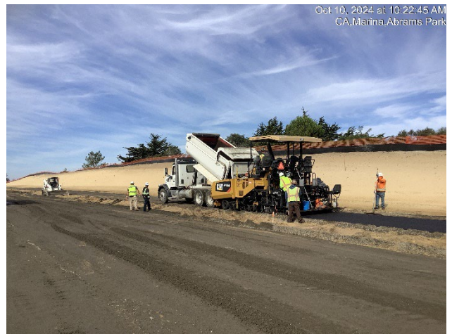
Paving bike path between Abrams and Marina Heights
