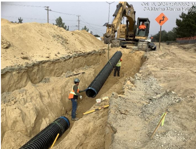
Installing storm drain at Imjin Road
