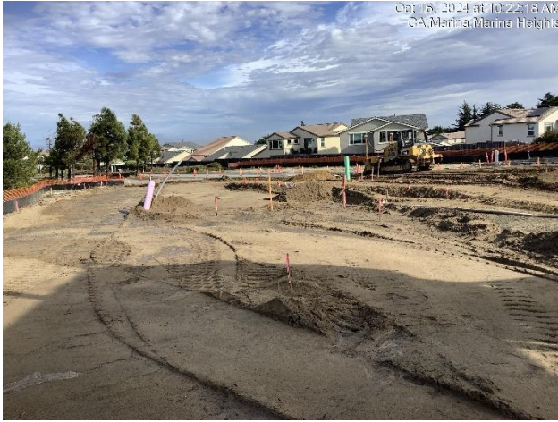
Marina Heights roadway grading
