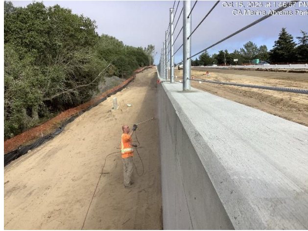
applying graffiti removal to concrete retaining walls
