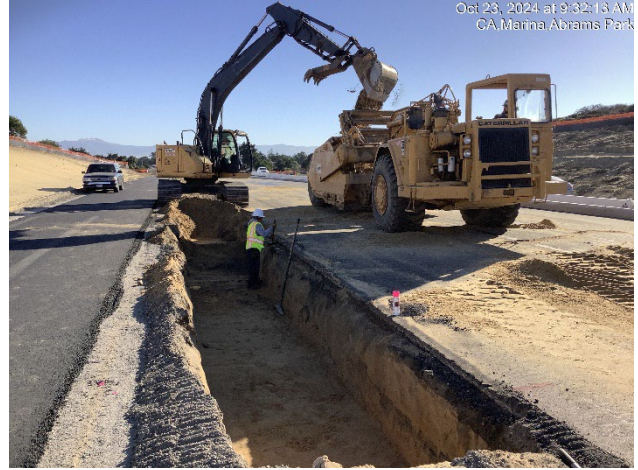
Construction of storm drain Bio retention for treatment storm runoff
