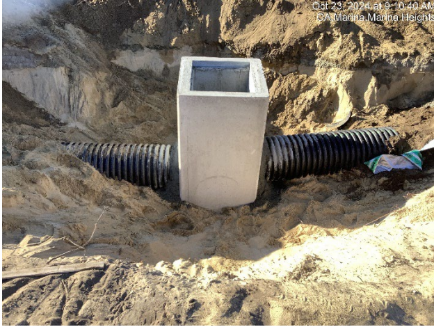
Construction of storm drain pipe and inlet at Imjin road
