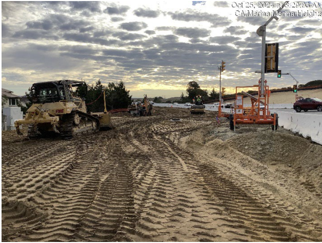
Construction of fill for roundabout at Imjin road
