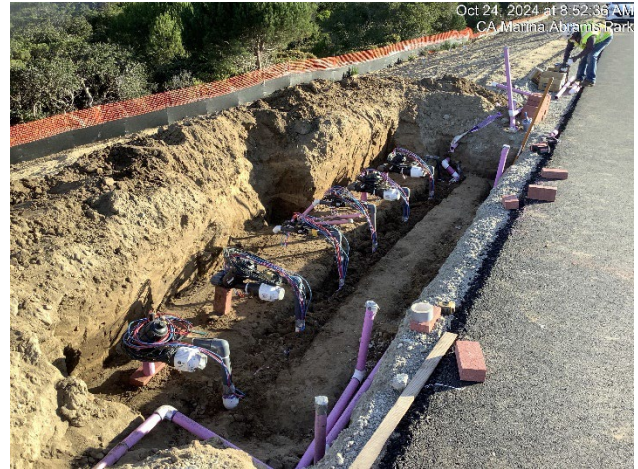
Construction of irrigation valves and piping
