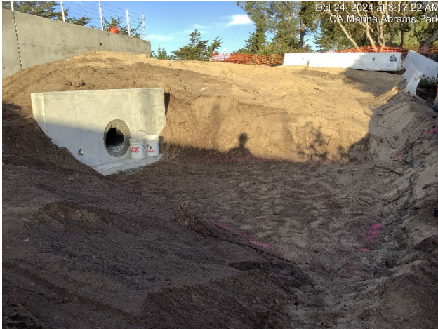
Construction of storm drain outlet through retaining wall at Abrams
