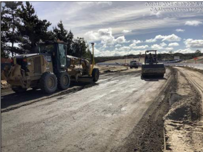
GRADING AND COMPACTING BASE MATERIAL FOR PHASE 1 ROADWAY NEAR IMJIN ROAD
