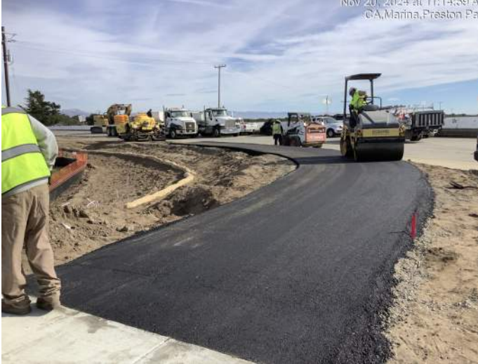
Temporary paving to connect sidewalk to bike path at Preston Drive
