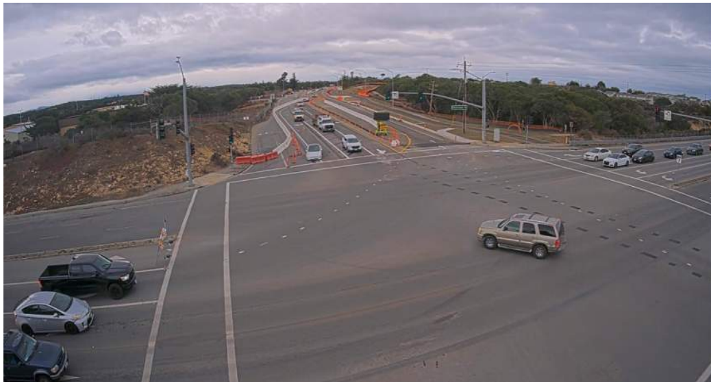
New lane configuration at Imjin Parkway/Reservation Road intersection
