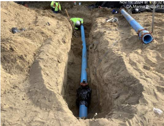
Domestic water service tie-in for Army Reserve and Chapin yard
