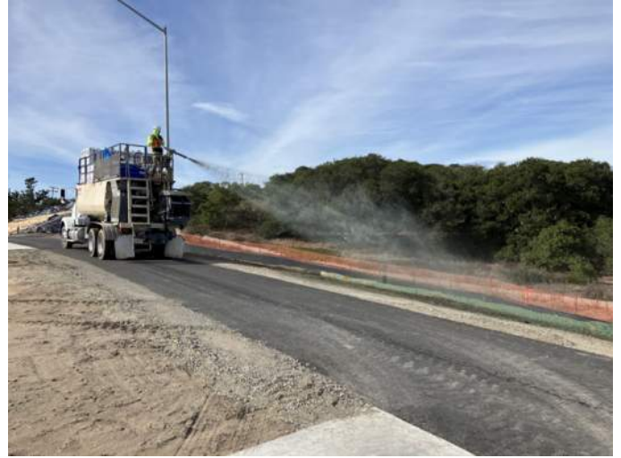
Hydroseeding slopes near Reservation Road
