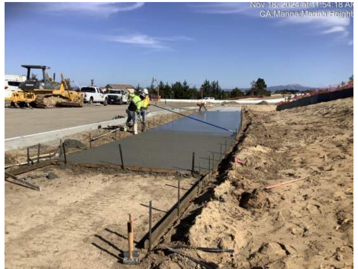
Concrete for sidewalk at Imjin Road
