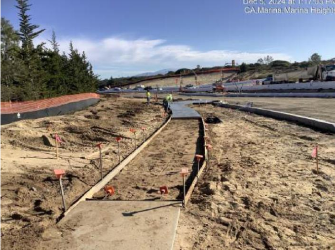
New sidewalk joins existing west of Imjin Road intersection
