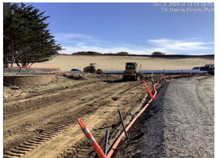
Grading and installation of fiber optic conduit along Marina Heights Drive
