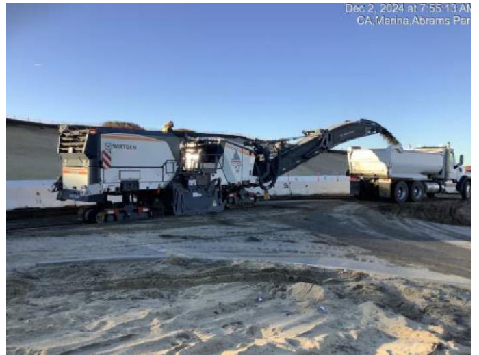
Grinding old pavement at Marina Height Drive
