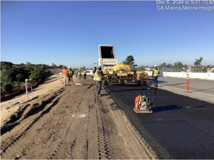
Temporary pavement along eastbound lane of Imjin Parkway.
