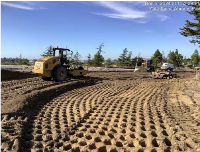
Grading and compaction west of Marina Heights Drive
