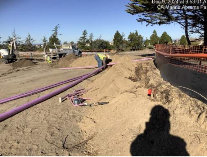
Installing irrigation pipe on Marina Heights Drive
