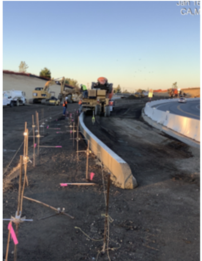
Extrusion machine extruding median curb along Imjin Parkway near Imjin Road
