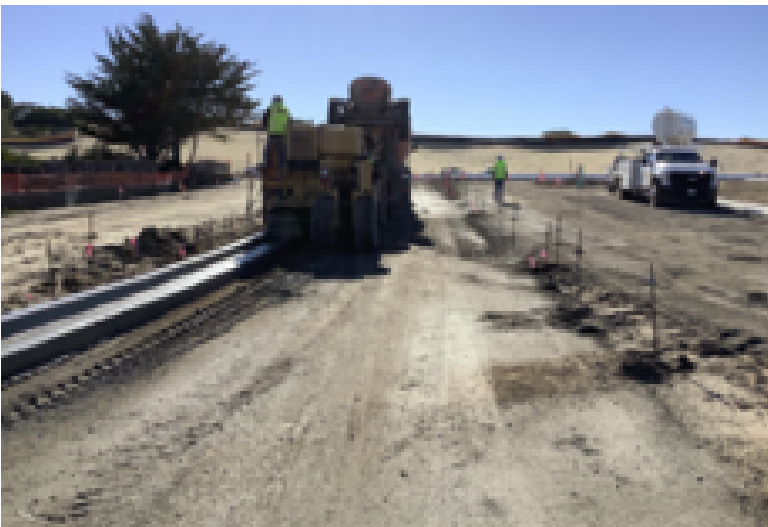
Extrusion machine extruding curb & gutter on Marina Heights Drive
