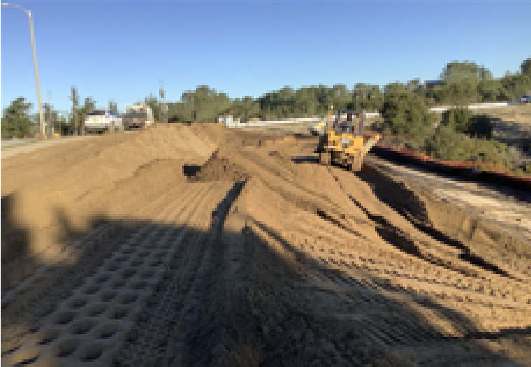
Embankment grading at SE Abrams Drive
