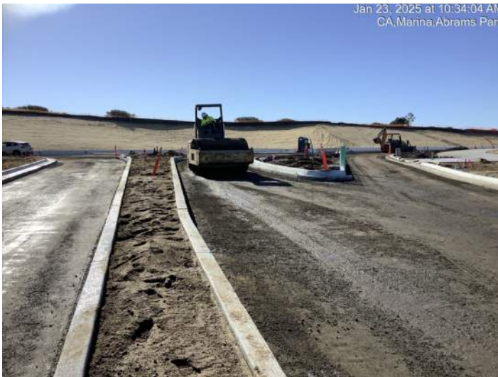
Compacting roadway base material on Marina Heights Drive
