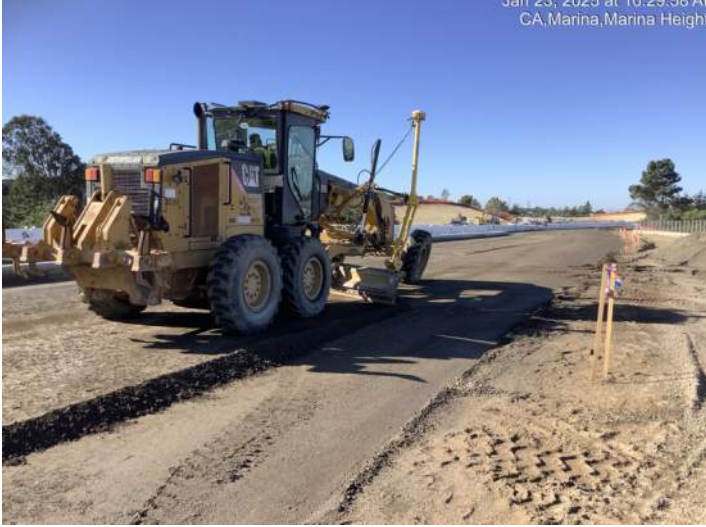
Fine grading between Marina Heights Drive and Imjin Road
