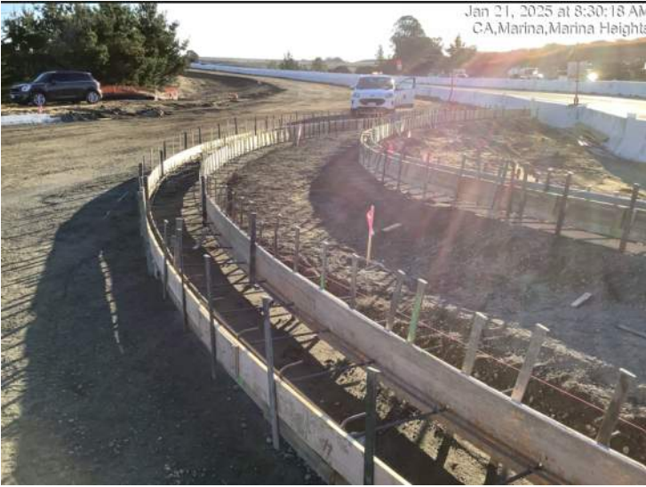
Formwork for 1/2 roundabout curb at Marina Heights Drive and Imjin Road
