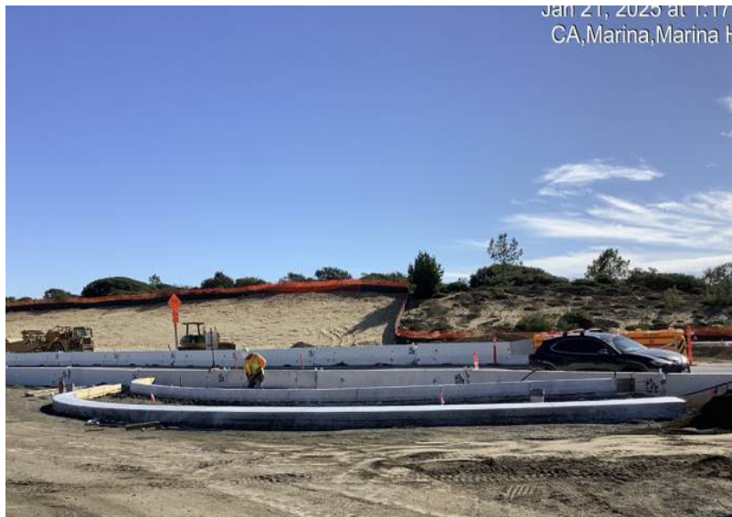
Concrete placed for 1/2 roundabout at Marina Heights Drive
