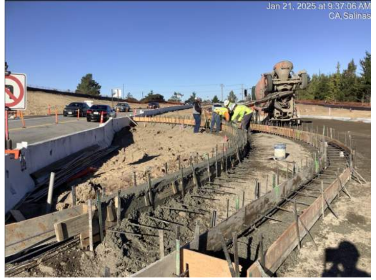
Formwork for 1/2 roundabout curb at Marina Heights Drive and Imjin Road
