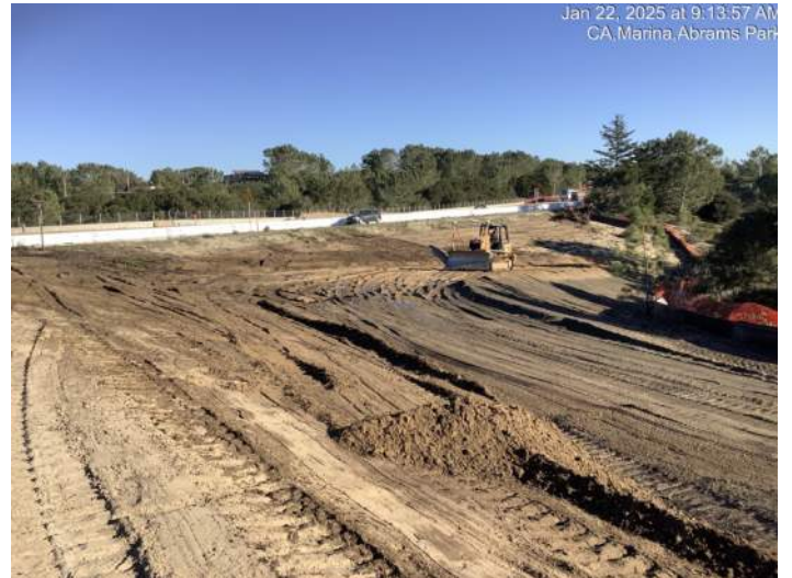
Embankment grading at SE corner of Abrams Drive
