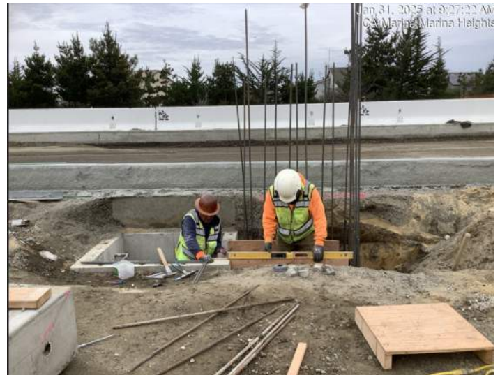
Forming drainage box for storm drain system near Imjin Road.
