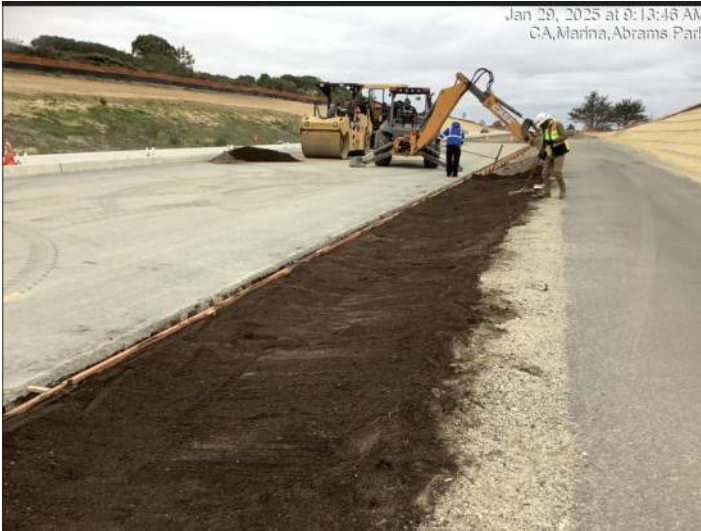
Installing special fill material for bio-retention basin(s) along Imjin Parkway
