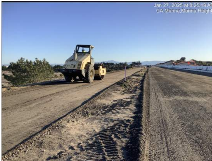
Finish grading work & compaction of materials under the bike/redestrian path.
