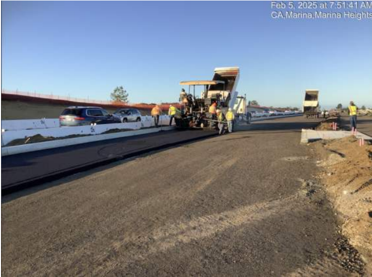
Paving operation for first lift of asphalt on Imjin Parkway westbound lanes - from western job limit (between Abrams Drive West and Imjin Road) to the 1/2 roundabout at Marina Heights Drive.
