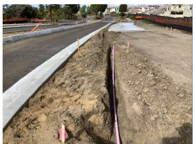
Installing irrigation service lines along Marina Heights Drive
