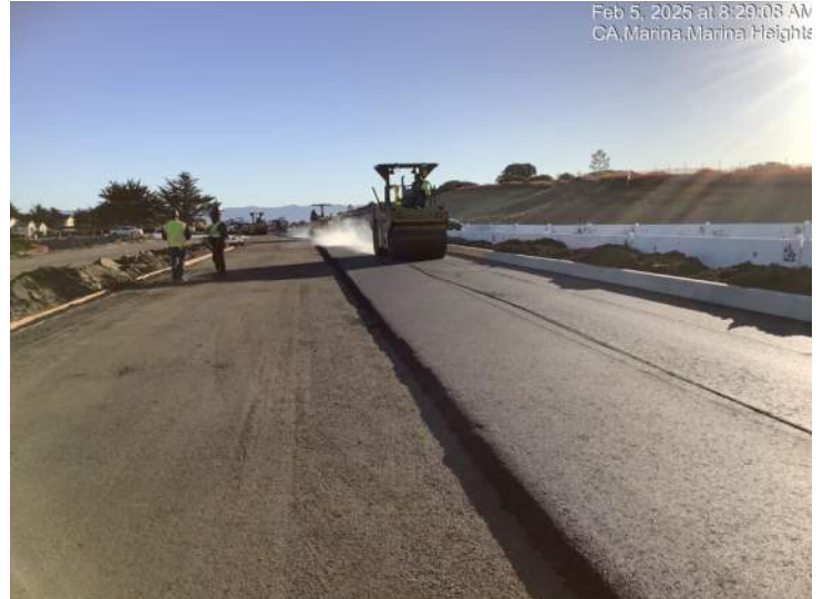
Paving operation for first lift of asphalt on Imjin Parkway westbound lanes - from western job limit (between Abrams Drive West and Imjin Road) to the 1/2 roundabout at Marina Heights Drive.
