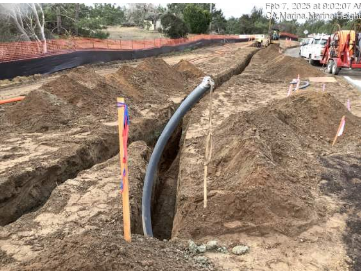
Installing electrical conduit for streetlights along Imjin Road
