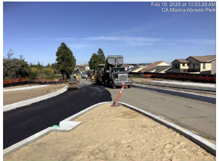
Paving first layer of asphalt for Marina Heights Drive
