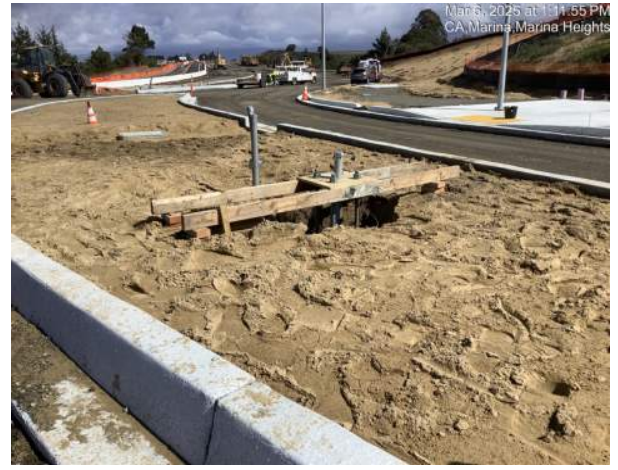
Street light foundation forms at Imjin Road
