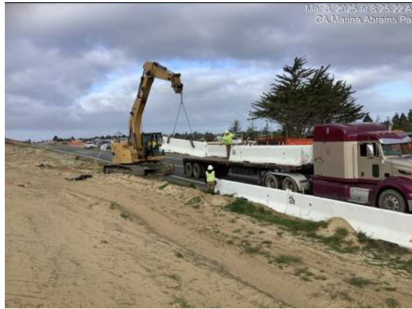
Loading out concrete barrier sections used in Phase 1
