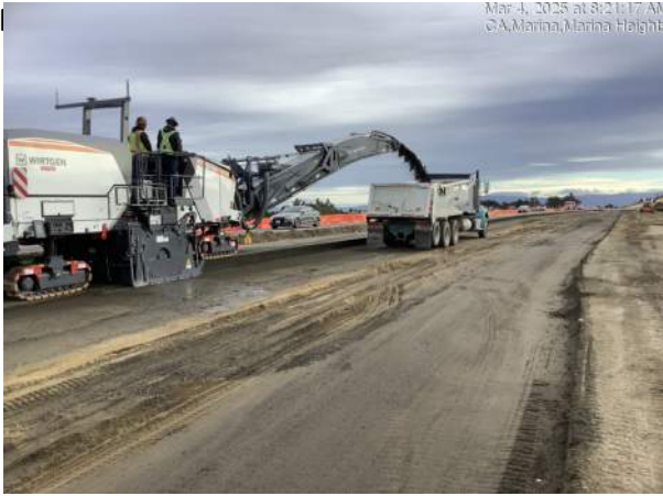
Grinding and removing existing roadway surface (south roadbed)
