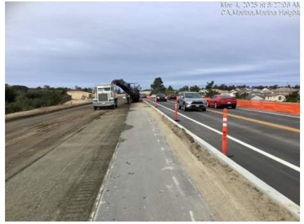
Grinding and removing existing roadway surface (south roadbed)
