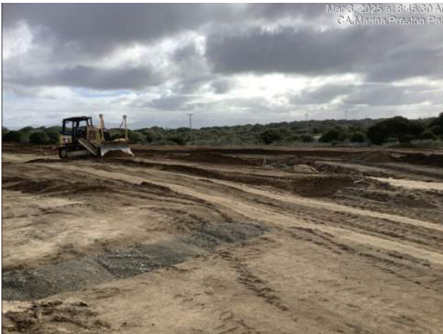
Grading operations across from Preston Drive
