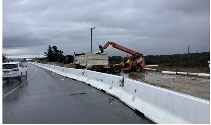
Removing abandoned sewer force main pipe at Preston
