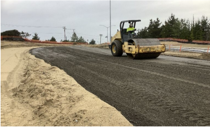
Grading and Base rock placement for roadway in Phase 2
