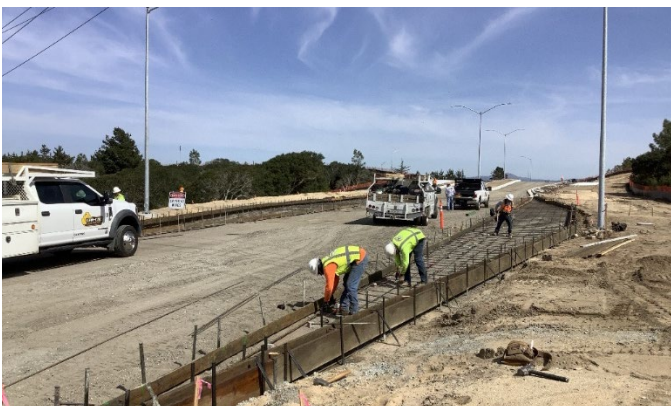
Forming for concrete sidewalk and bus pad at Imjin Road
