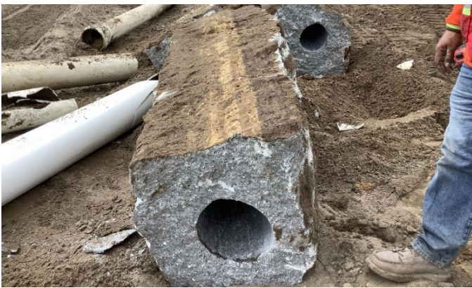
Removed abandoned sewer force main pipe
