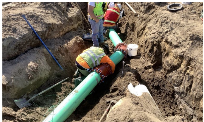
New relocated sewer force main pipe
