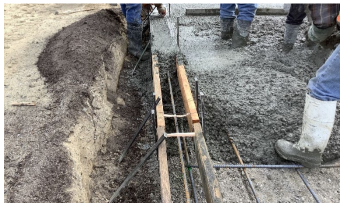
Installing concrete sidewalk and bus pad at Imjin Road
