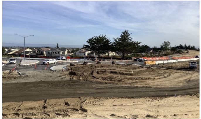
Marina roundabout medium being graded
