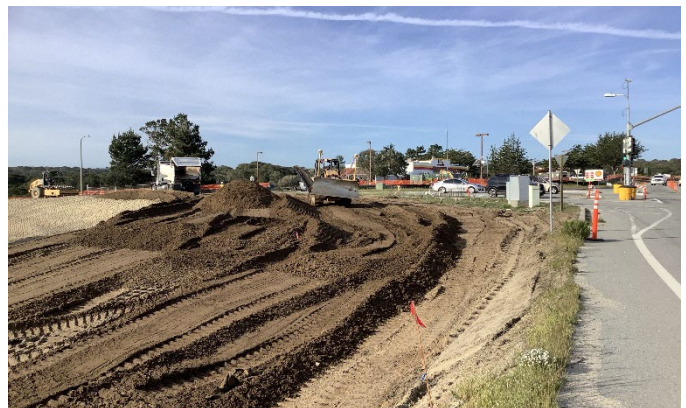
Abrams south side embankment fill being placed
