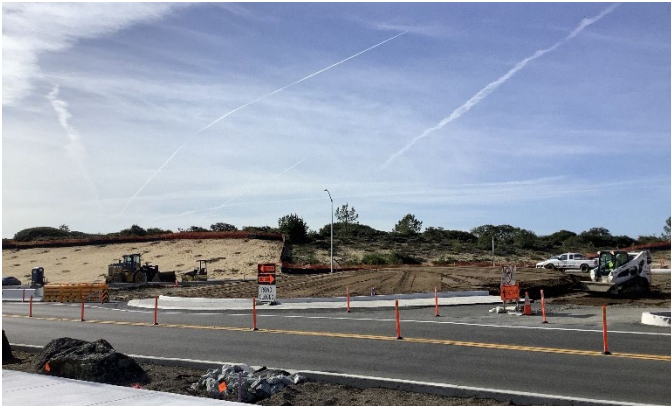
Imjin Rd roundabout medium being graded
