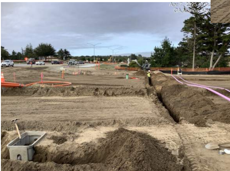
Trenching and installing irrigation service lines at Abrams Drive (north side)
