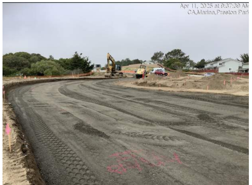
Grading base rock for roadway section at Preston Drive roundabout area
