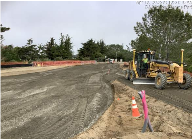
Grading operations at Abrams Drive (north side)
