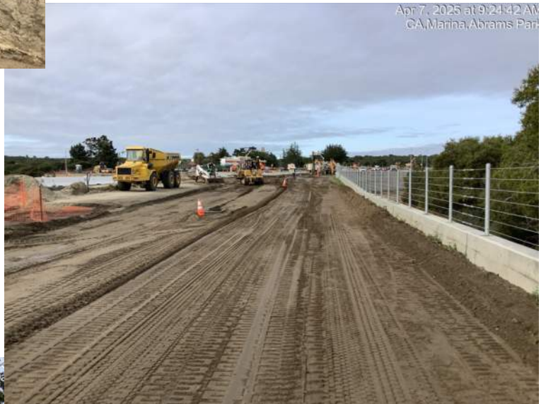
Grading operations at Abrams Drive (north side)
