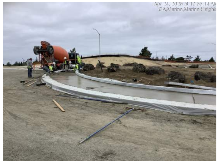
Placing concrete for truck apron at Imjin Road roundabout
