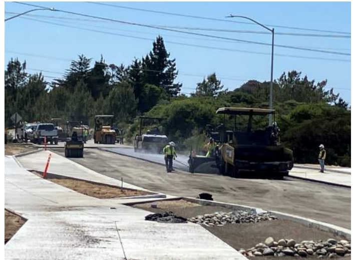
Paving first layer of asphalt at Imjin Road
