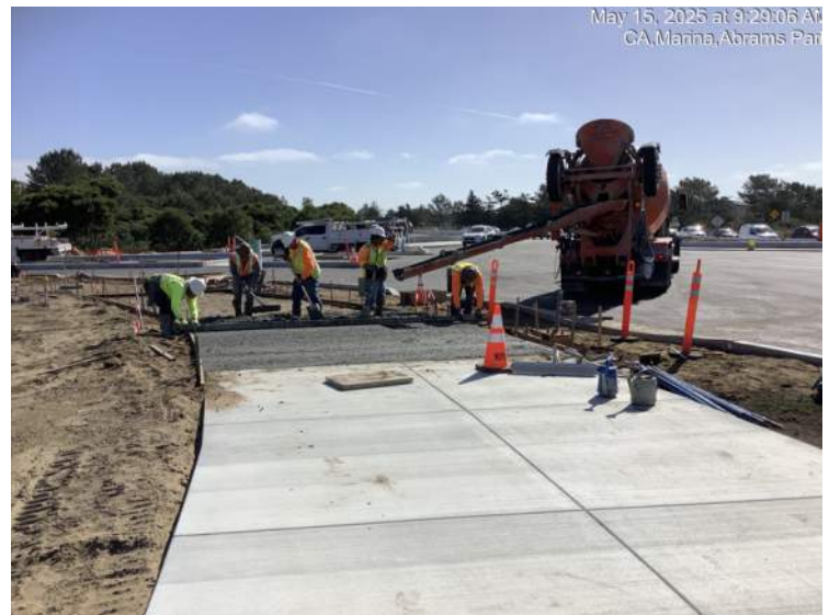
Placing concrete for sidewalks at Abrams Drive (north)
