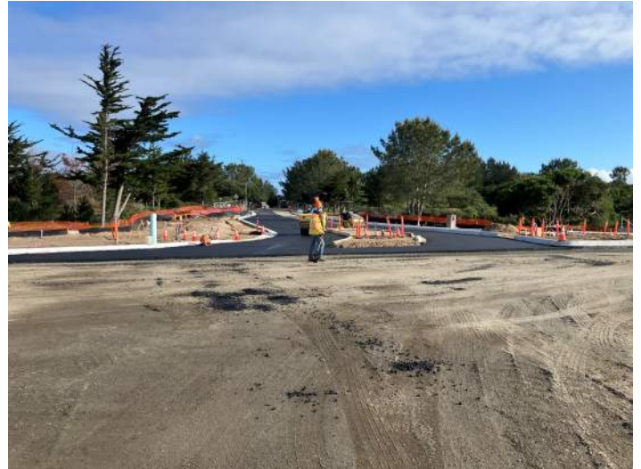
Paving first layer of asphalt at Abrams Drive (north)
