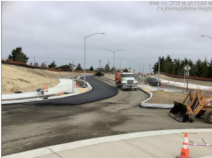
Paving first layer of asphalt at Imjin Road
