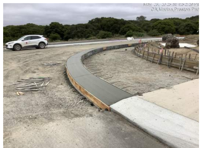
Concrete placed for curbs at Preston Drive roundabout
