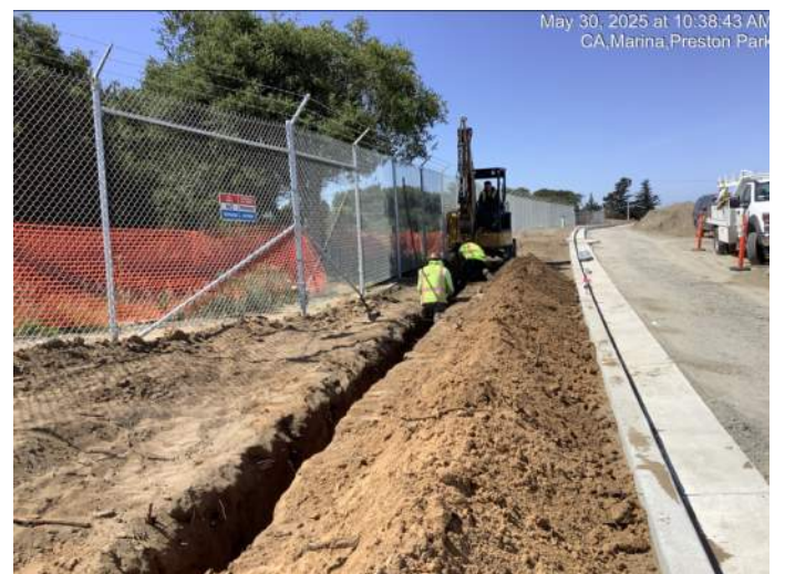
Trenching for installation of electrical conduits
