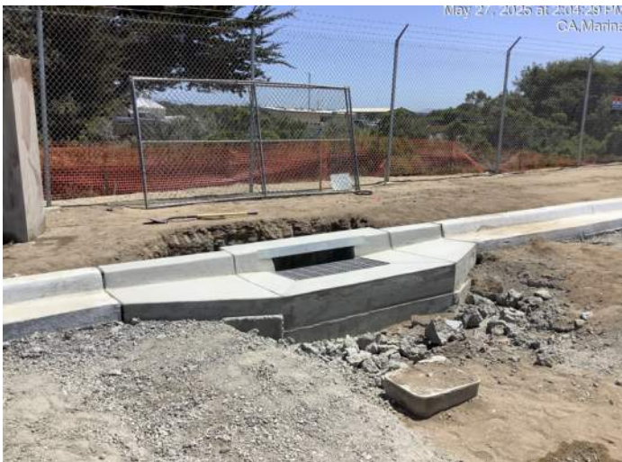
Storm drain inlet near the Army Reserve
