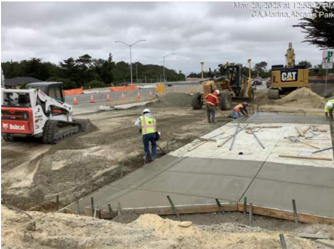
Placing concrete for "wings" of new driveway at the Shell station
