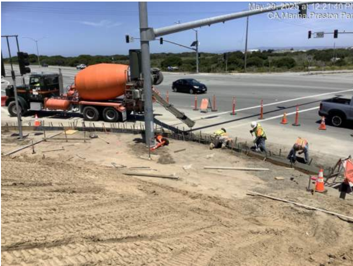
Placing concrete for curb & gutter at ImjinPkwy/Reservation Rd.
