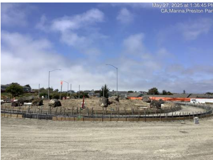
Forming for curbs at Preston Drive roundabout
