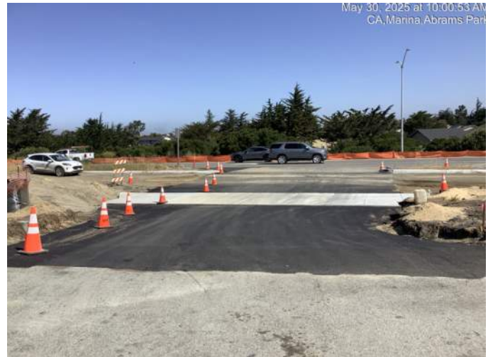
Asphalt installed to tie in new driveway at the Shell station
