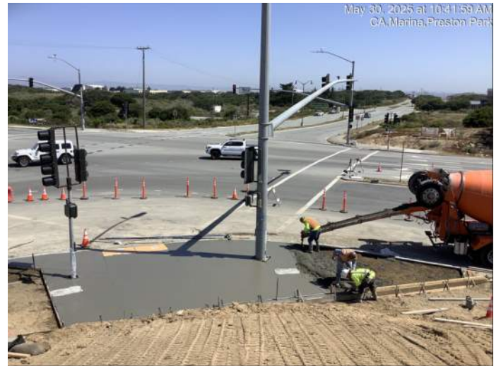
Placing sidewalk concrete at ImjinPkwy/Reservation Rd.
