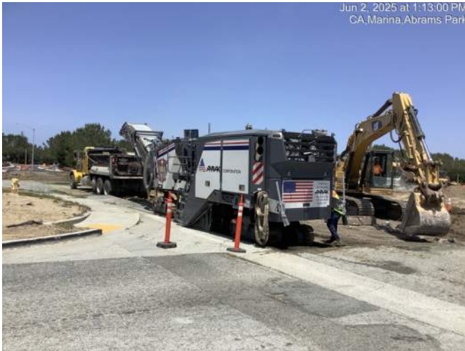
Grinding and removal of existing pavement for the south roadway section between Shell station driveway and Chapin driveway
