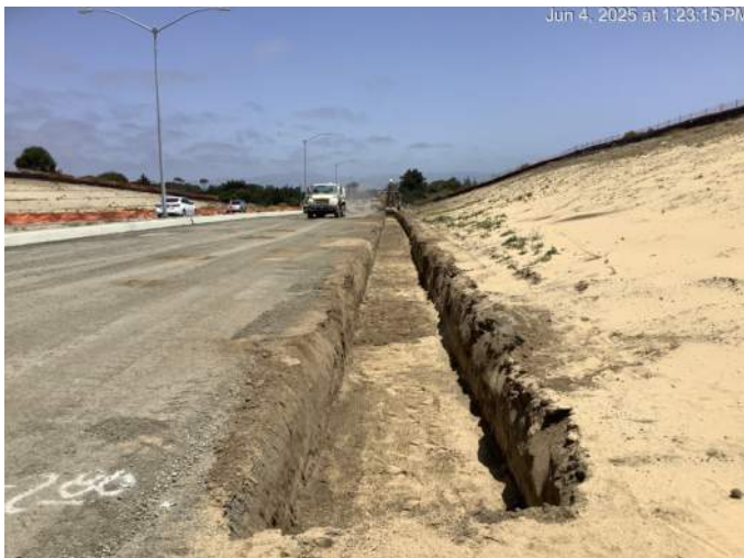
Trench for installation of bio swale materials
