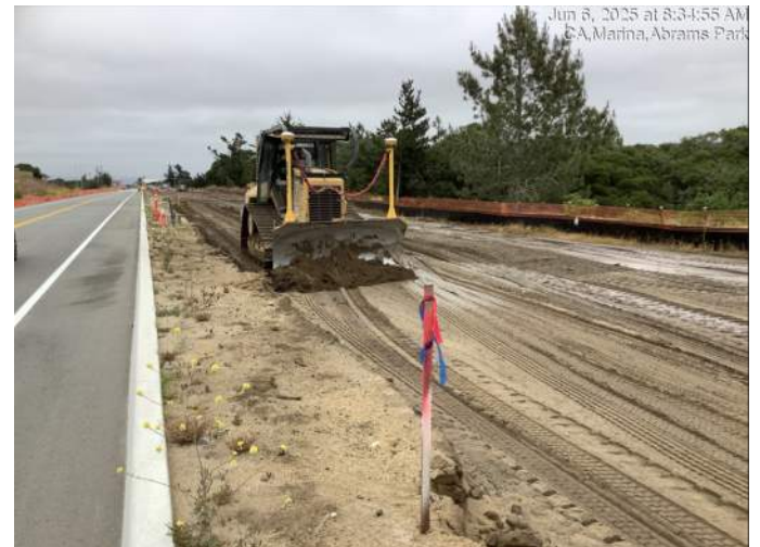
Earthwork/grading for the south roadway section between Shell station driveway and Chapin driveway
