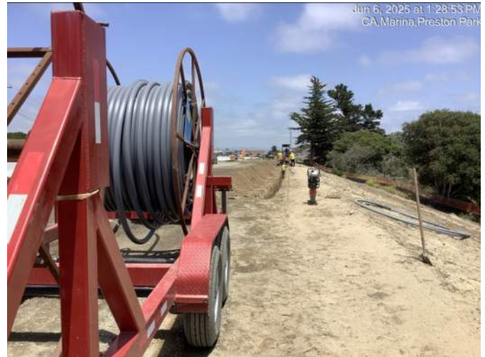
Installing electrical conduit between Chapin driveway and Preston Drive
