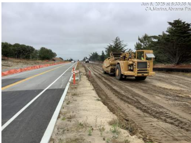
Earthwork/grading for the south roadway section between Shell station driveway and Chapin driveway
