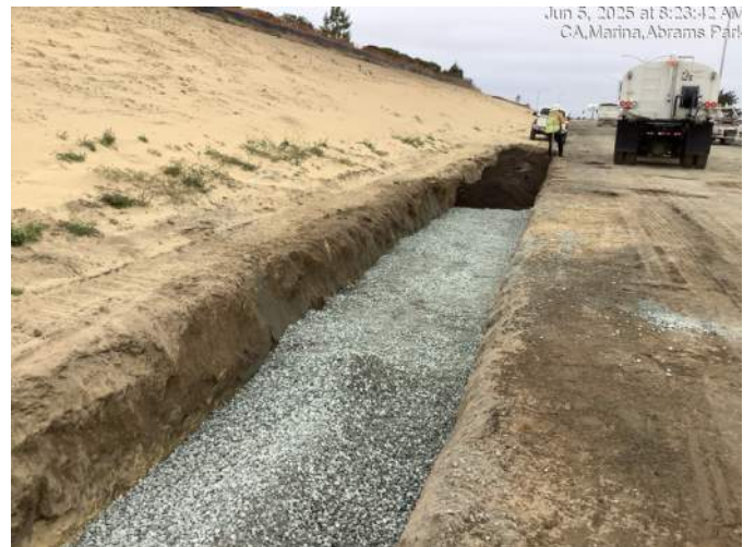
Drain rock (gray) followed by specialty soil material (darker material) for bio swale
