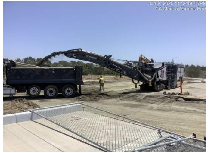
Grinding and removal of existing pavement for the south roadway section between Shell station driveway and Chapin driveway
