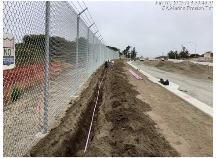
Installing irrigation services lines near Reservation Road
