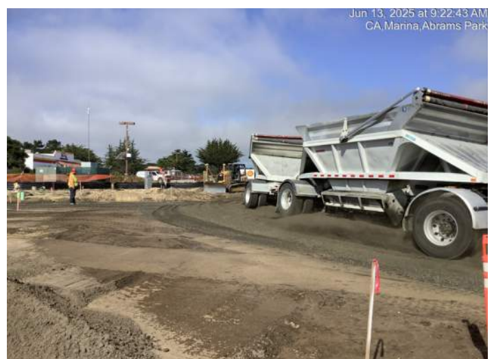
Based rock delivery at SE corner of Abrams Drive (south)
