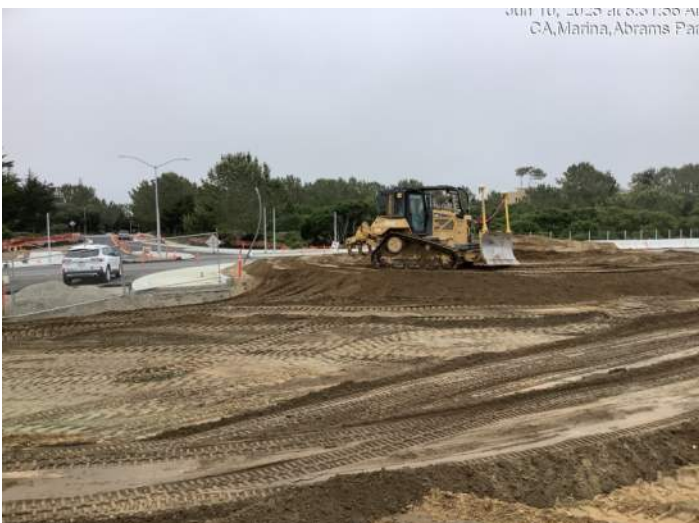
Grading for the south half of roundabout at Abrams Drive
