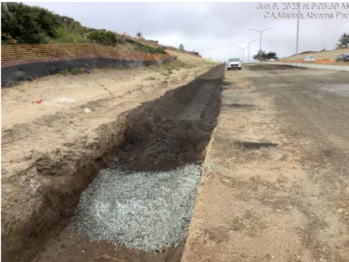
Installing materials for bioswales between Marina Heights Drive and Shell station driveway
