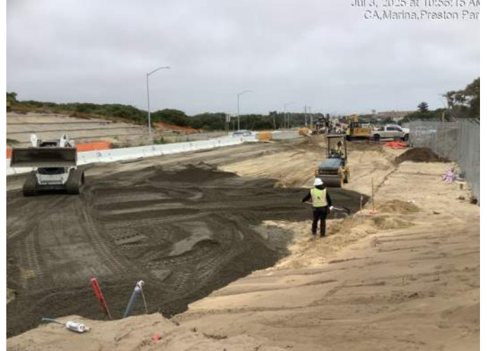
Placing base rock (layer under the asphalt) near the Army Reserve
