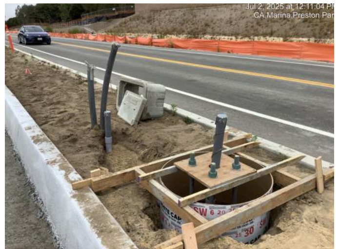
Forming for median street light foundation (along Imjin Parkway)
