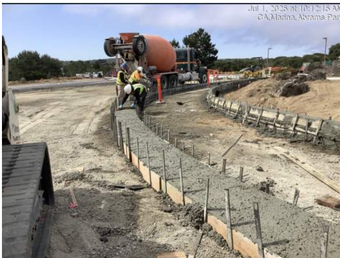
Placing concrete for outer curb of roundabout at Abrams Drive (south)
