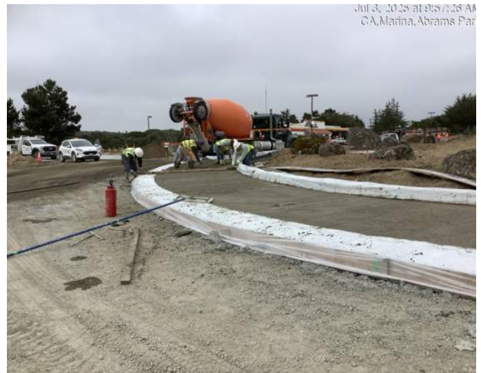
Placing concrete for inside "truck apron" of roundabout at Abrams Drive (south)
