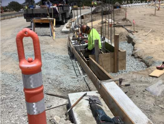
Forming drainage inlet at Abrams Drive (south)
