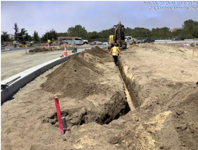
Trenching for electrical conduit at Abrams Drive (south)
