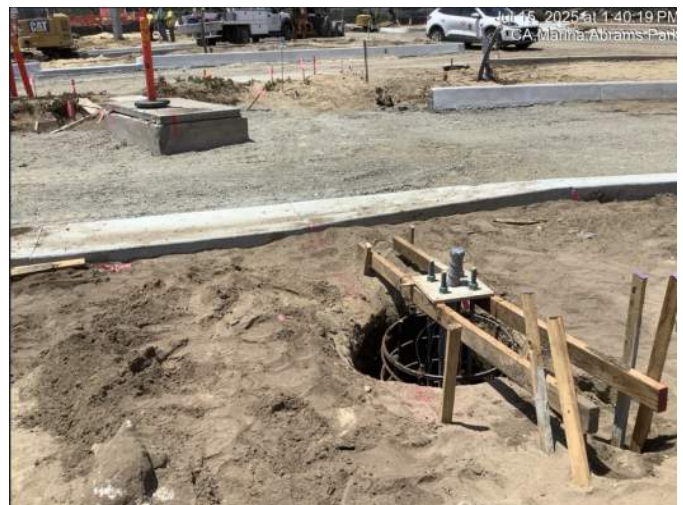
Street light foundation formed at Abrams Drive (south)
