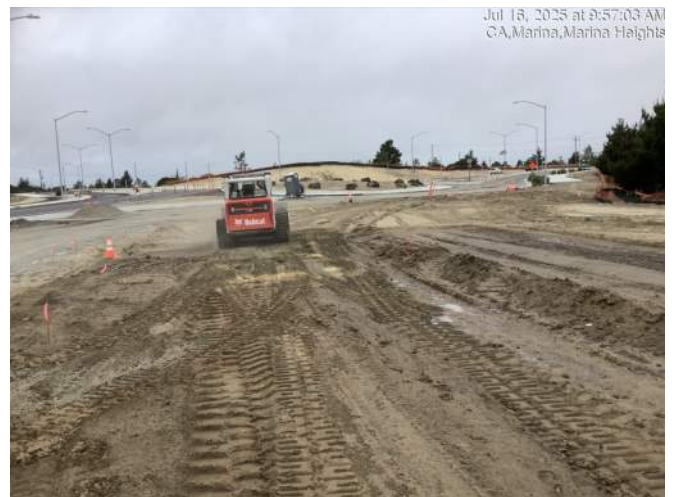
Rough grading for Imjin Parkway (north roadbed) near Imjin Road
