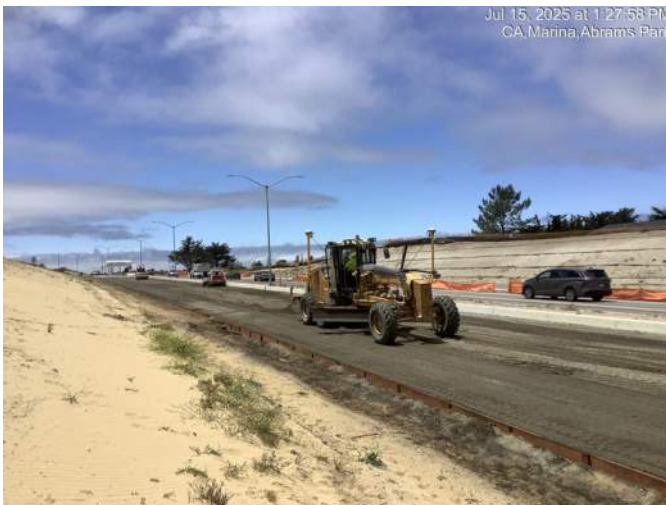
Final grading work on Imjin Parkway (south roadbed)
