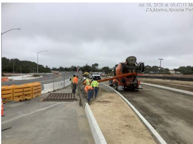
Placing concrete for median curb "tie-in" near Abrams Drive (south)
