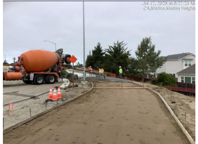
Placing concrete for sidewalk concrete near Imjin Road
