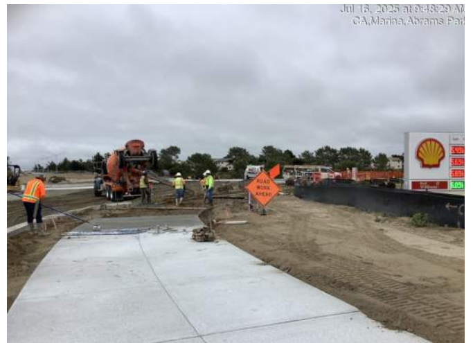
Placing concrete for sidewalk at Abrams Drive (south)
