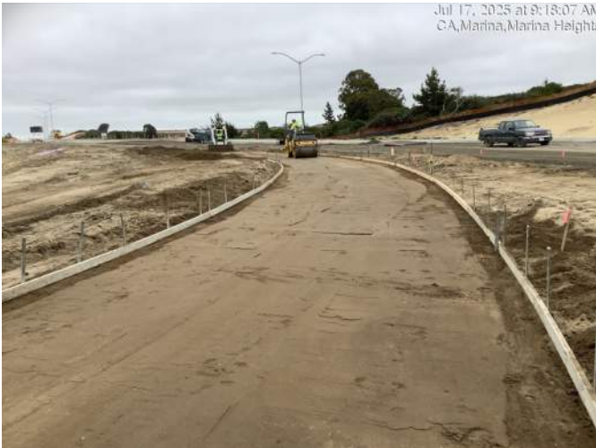
Preparing subgrade material for sidewalk concrete near Imjin Road
