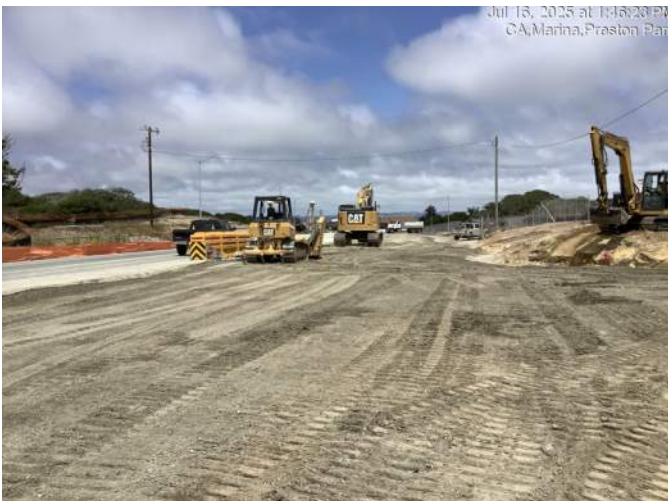
Rough grading for Imjin Parkway (south roadbed) near the Army Reserve
