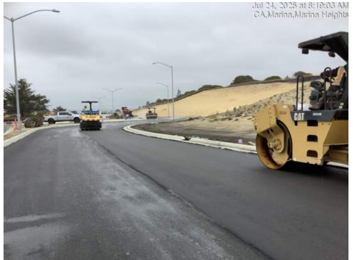
Paving first layer of asphalt for the south roadbed (near Marina Heights Drive)
