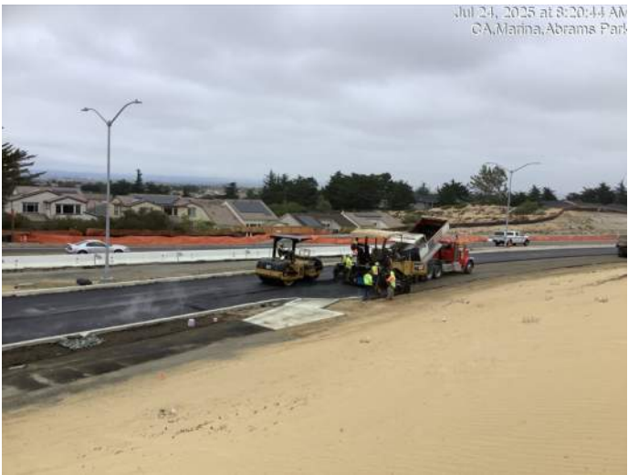
Paving first layer of asphalt for the south roadbed (near Imjin Road)
