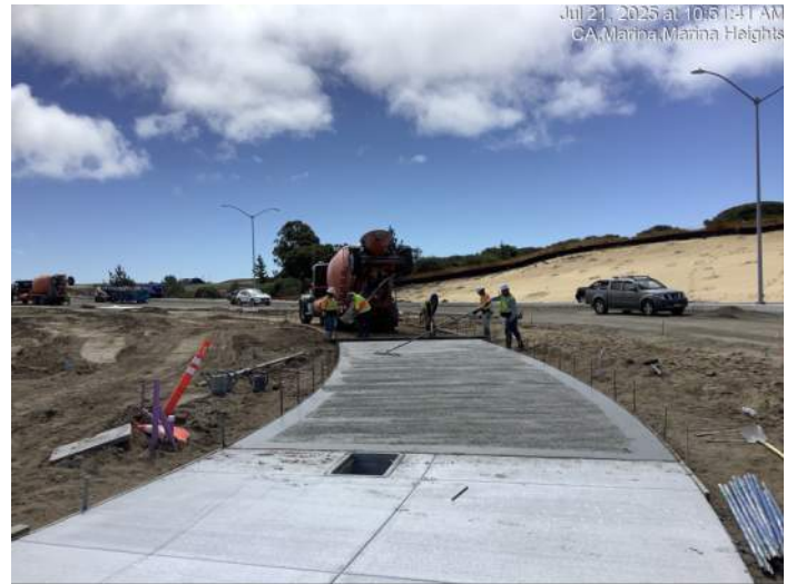
Placing concrete for sidewalk near Imjin Road
