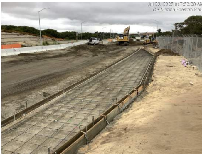
Forms and reinforcing steel for bus pad near Army Reserve
