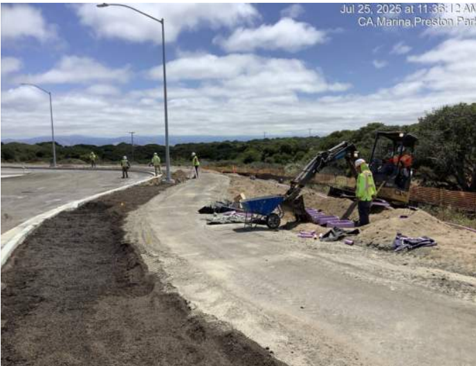
Installing irrigation elements (purple pipe = recycled water use)
