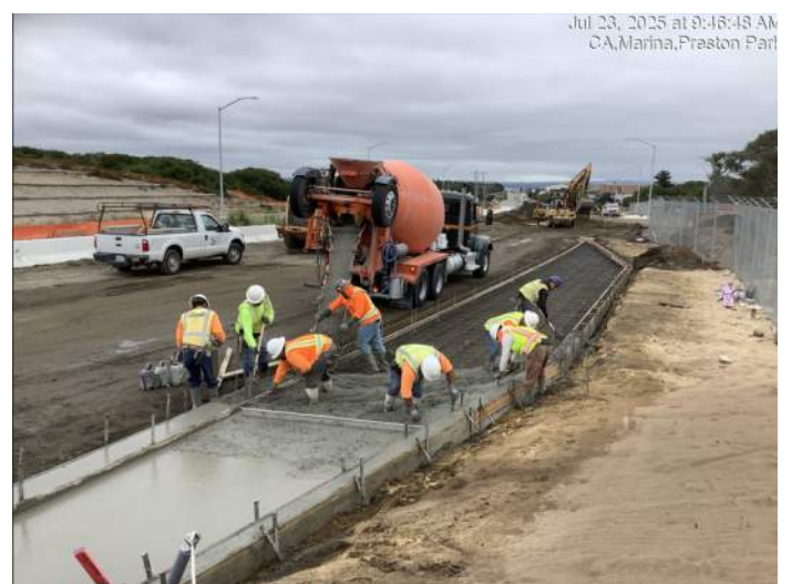
Placing concrete for bus pad near Army Reserve
