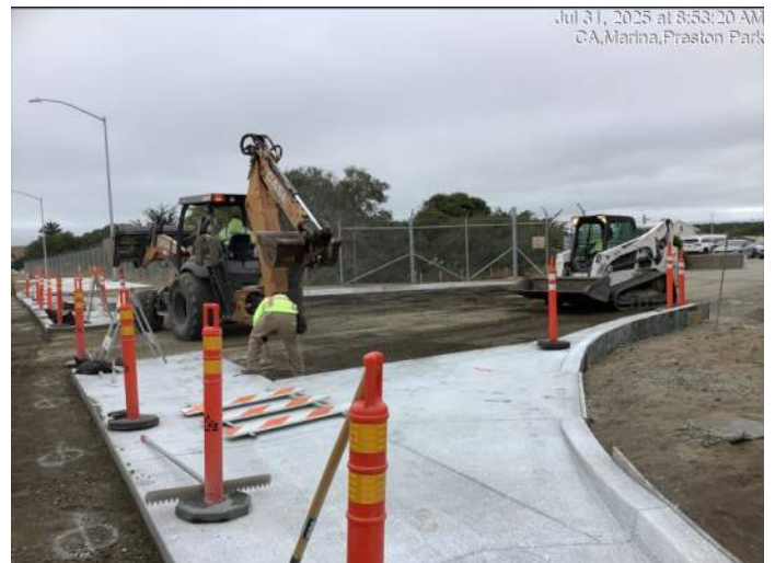
Grading for asphalt portion of the Army Reserve driveway
