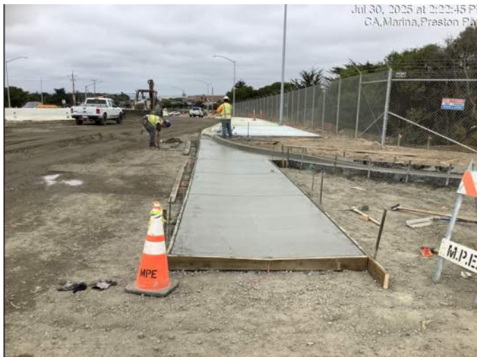
Portion of concrete cross gutter at the Army Reserve driveway
