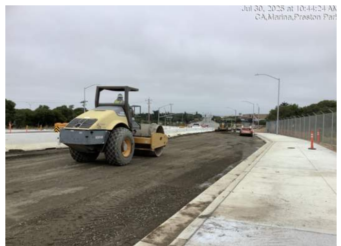
Fine grading of base materials for south side of Imjin Parkway
