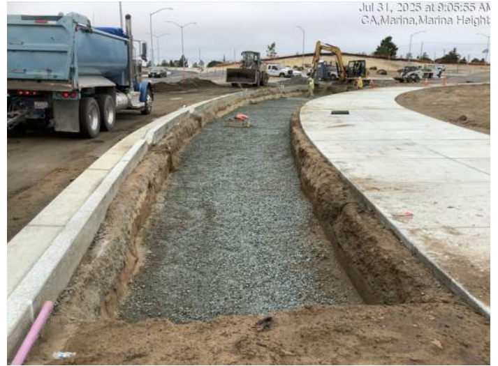
Installation of drain rock for bioswale near Imjin Road
