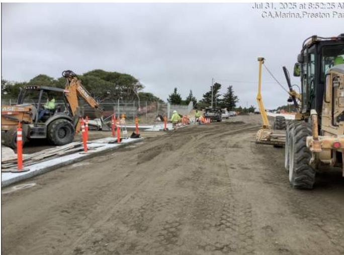
Fine grading of base materials for south side of Imjin Parkway
