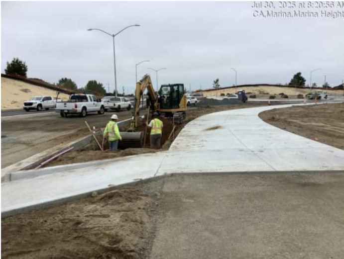
Excavation of soils for bioswale near Imjin Road
