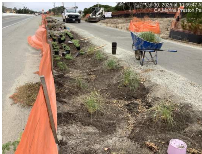
Installation of native plants for bioswale approaching Preston Drive
