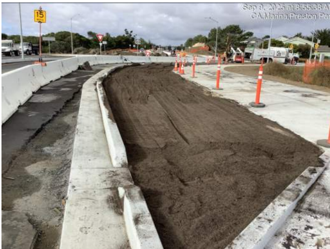
Bioswale material (dark colored soil) installed near Abrams Drive (north)
