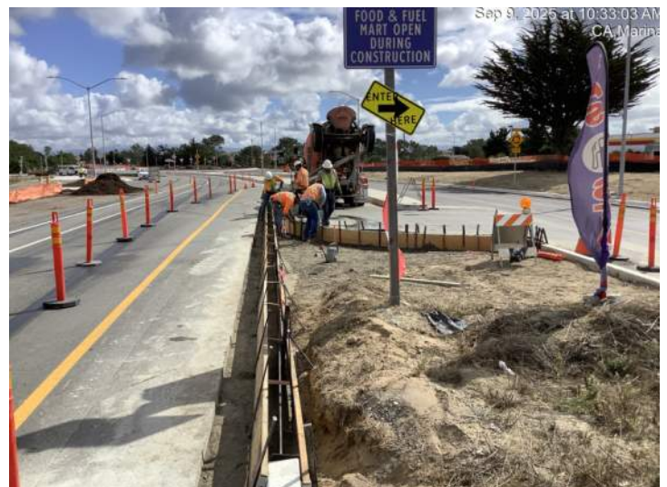
Placing concrete median curb at left turn pocket for food & fuel mart
