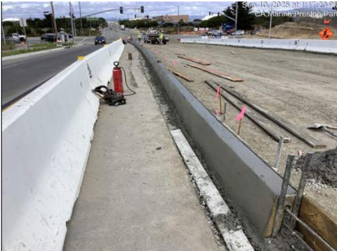
Placing concrete for median curb between Army Reserve and Reservation Road
