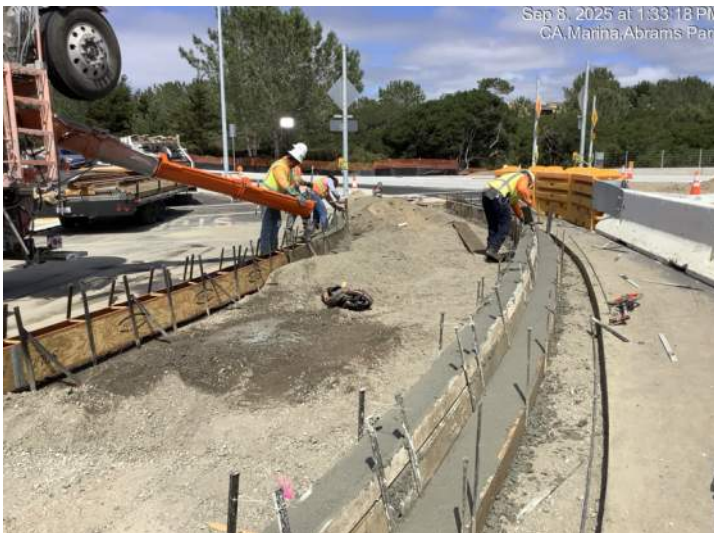
Placing concrete for splitter island curb & gutter at Abrams Drive (north)
