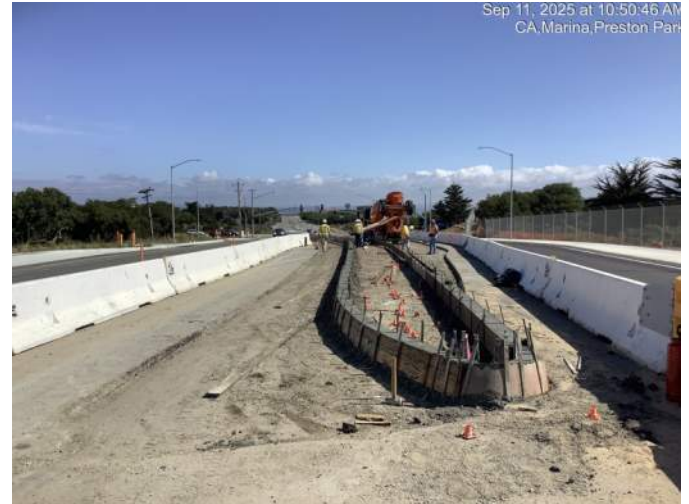
Placing concrete for median curb between Army Reserve and Reservation Road
