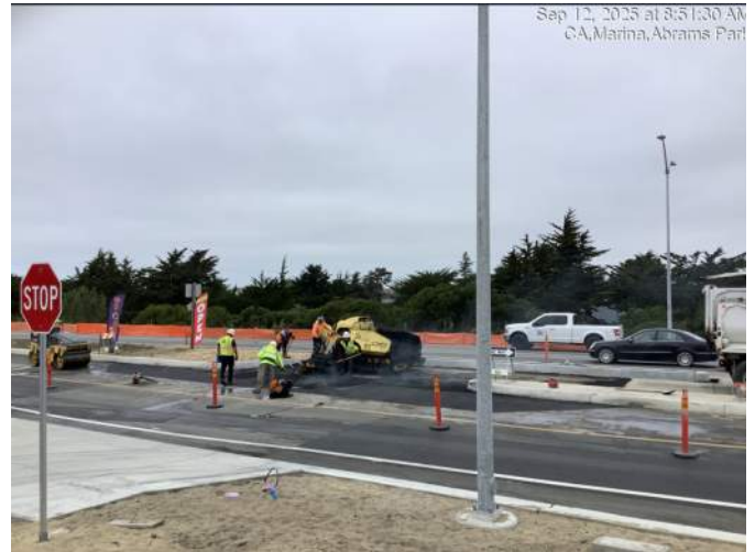
Paving first layer of asphalt at left turn pocket for food & fuel mart
