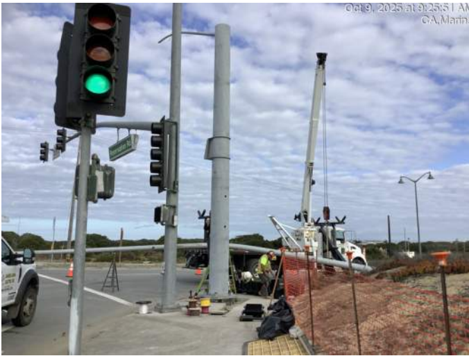
Standing new signal pole at Imjin Road/Reservation Road
