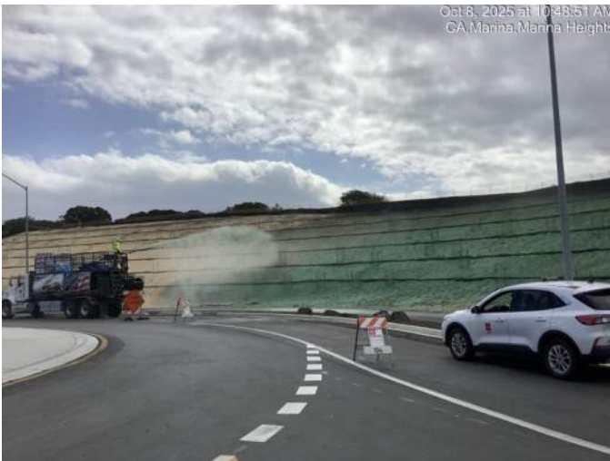
Hydroseeding slope at Imjin Road
