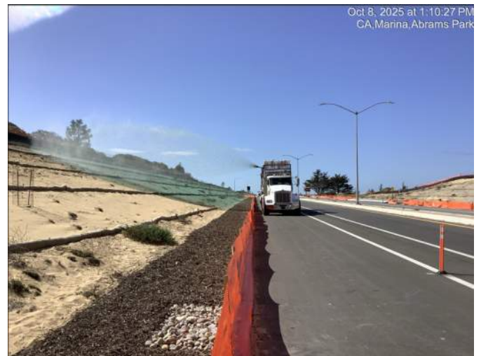
Hydroseeding slope near Marina Heights Drive
