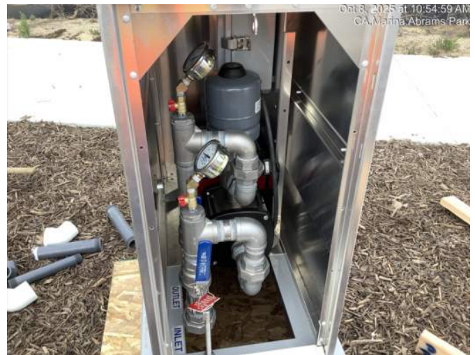
New booster pump to provide additional line pressure for plant establishment irrigation on slopes near Marian Heights Drive
