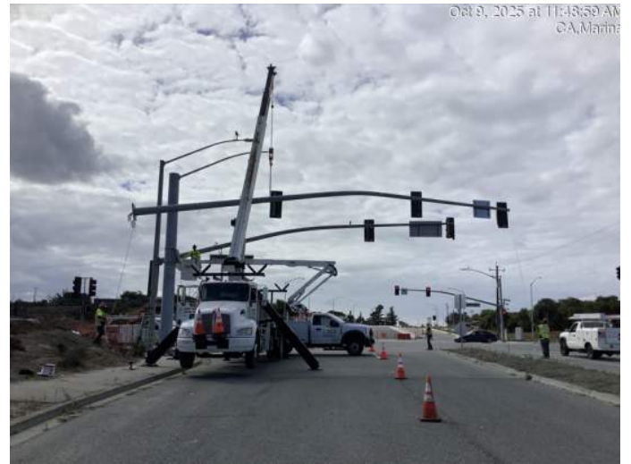
Installing arm on new signal pole at Imjin Road/Reservation Road
