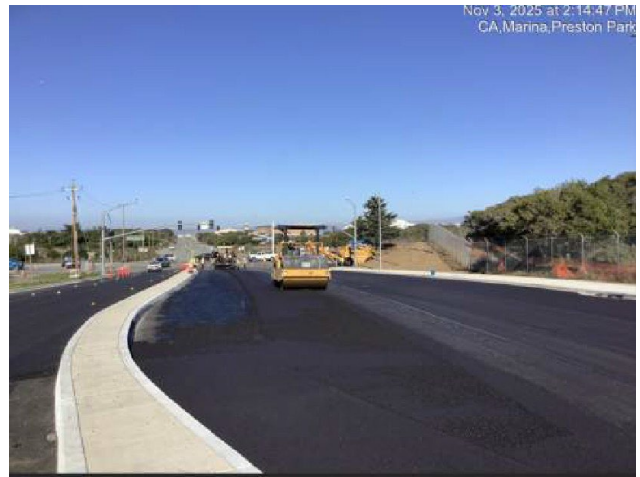
Final lift (layer) of paving on Imijn Parkway between Army Reserve and Reservation Road
