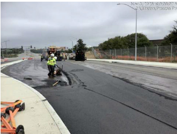
Final lift (layer) of paving on Imijn Parkway between Army Reserve and Reservation Road
