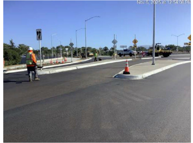
Final lift of paving on Abrams Drive (north)
