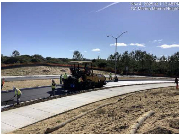
Final lift (layer) of paving on Imijn Parkway between Army Reserve and Reservation Road
