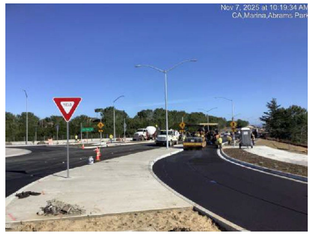
Final lift of paving on Abrams Drive (south)
