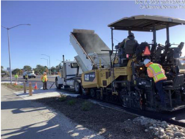
Final lift of paving on Abrams Drive (north)
