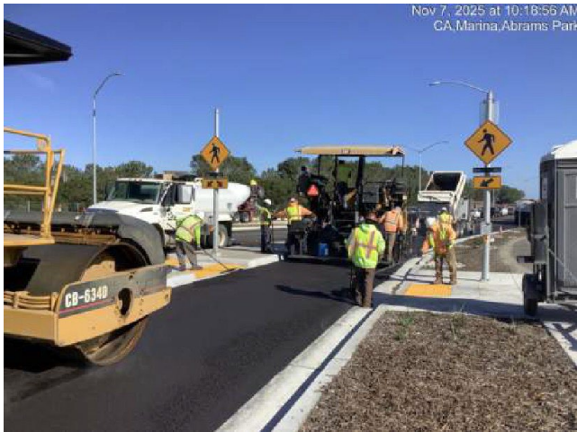
Final lift of paving on Abrams Drive (south)
