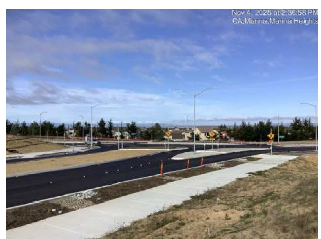
Final lift (layer) of paving on Imijn Parkway between Army Reserve and Reservation Road
